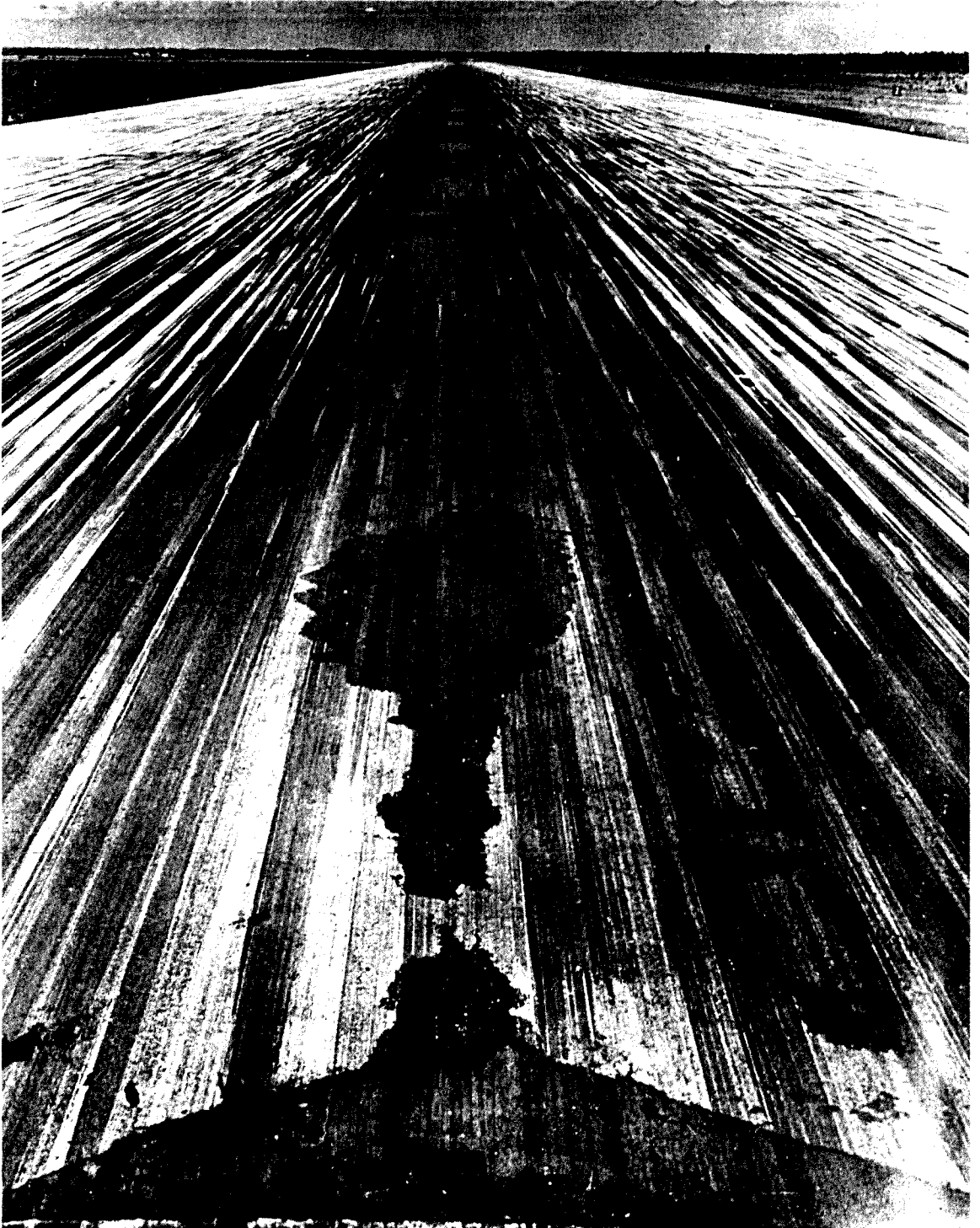
Fig. 2. Effects of concentration of traffic in the central 20 ft of runway at Pinecastle AFB
