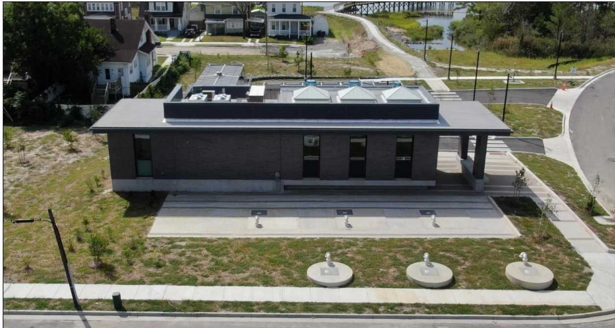
Figure 7. Aerial view of the Ballentine Pump Station designed to fit with the historic character of the neighborhood. The pump station includes features such as publicly accessible power outlets, parking, and sheltered space from the elements. The pump station is designed to handle increased amounts of rainfall today and into the future. Image courtesy of the City of Norfolk.
