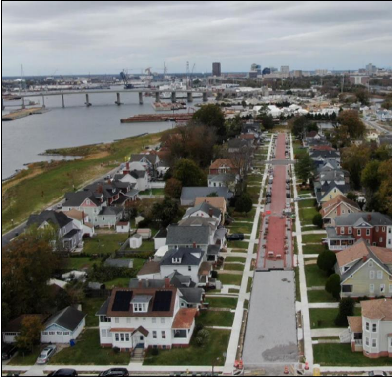
Figure 6. Aerial view of the pervious pavers (red colored) being placed on Marlboro Avenue in the Chesterfield Heights neighborhood. Image courtesy of the City of Norfolk.
