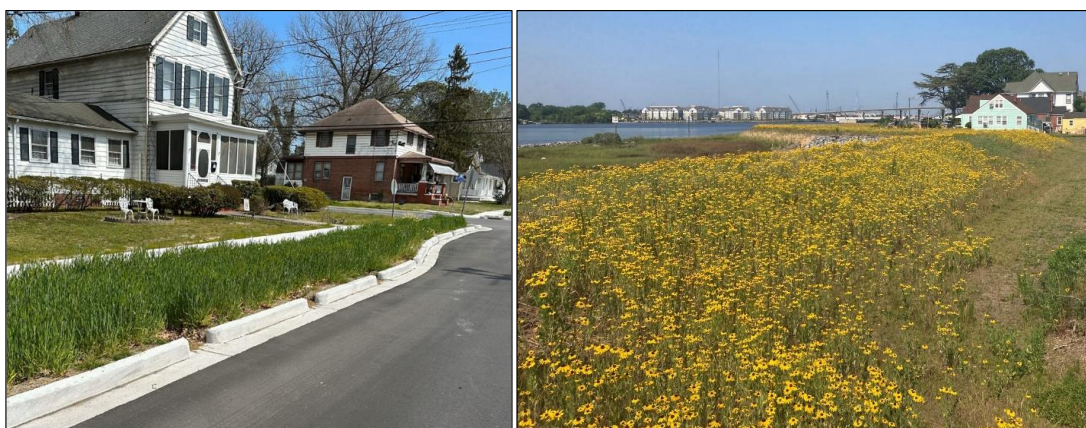
Figure 3. Neighborhood bioswales were installed and planted with native species as a localized flood risk reduction measure while also providing groundwater infiltration and habitat uplift benefits ( left ). The earthen berm constructed to reduce flood risk was planted with native wildflower species to enhance the habitat value associated with the structure ( right ). Images courtesy of the City of Norfolk.
