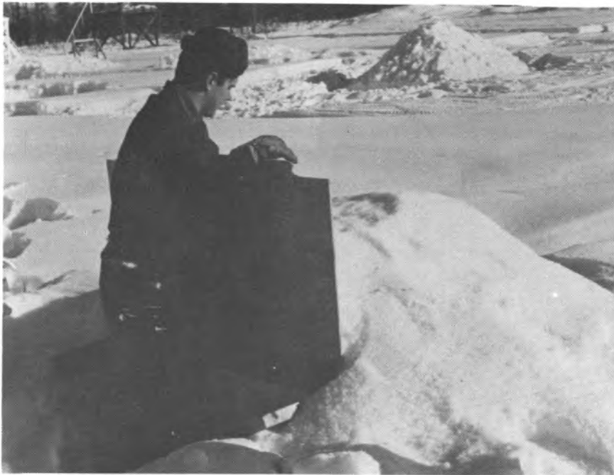
Figure 27. Snow arch form in use.
