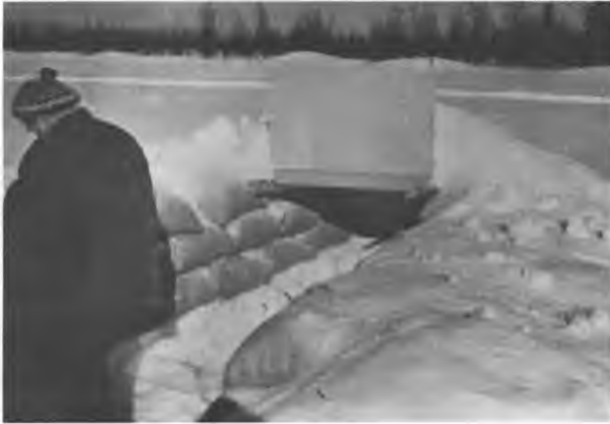
Figure 20. Snow trench revetted with snow bags.
