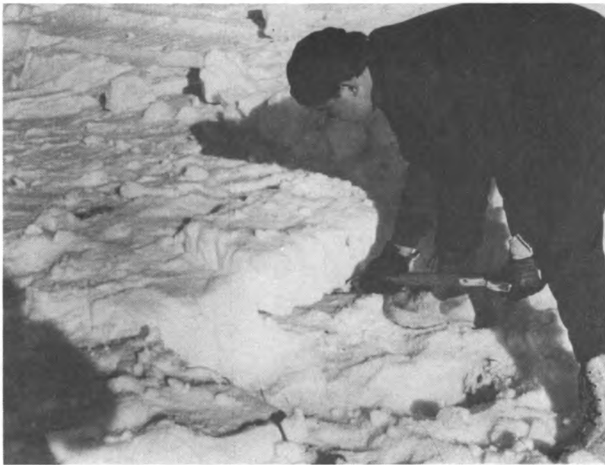
Figure 22. Mining a snow block in packed snow.
