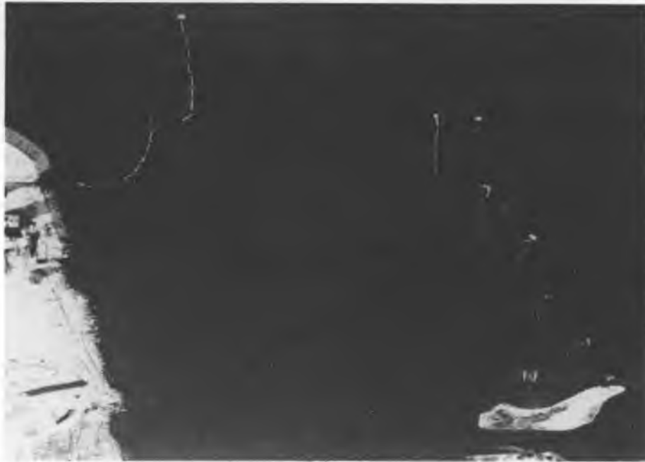
Figure 8. Aerial view of installed ice booms, looking downstream along course 2, St. Marys River, Michigan, 23 December 1975.
