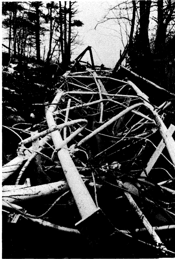
Figure 1. Wreckage of WCSH-TV's (Portland, Maine) 1300-foot tower felled by severe icing on 9 March 1983.
