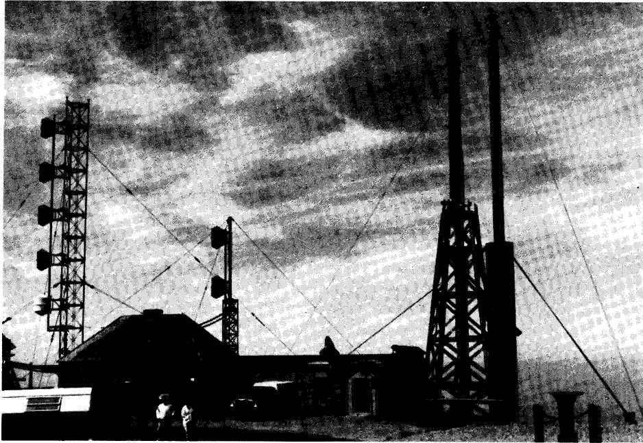
Figure 3. Radio and TV towers at the summit of Mt. Washington. WMTW-TV's tower, shown at extreme right, is radome-enclosed and less prone to icing than their old tower with exposed framework.
