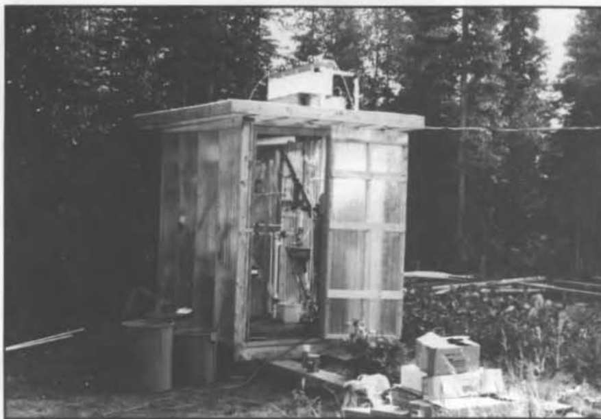
Figure 4. Pilot plant building.
