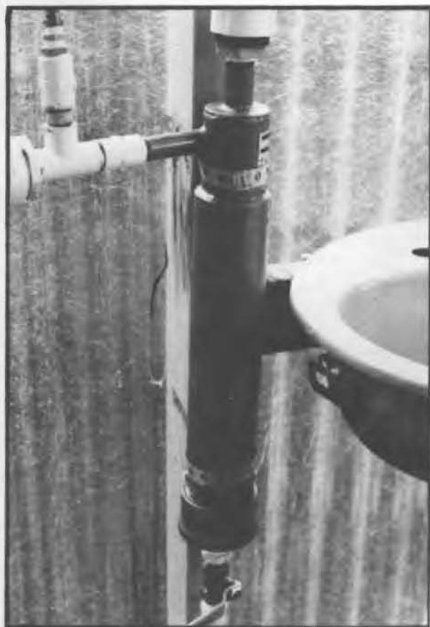
Figure 6. Hydrocyclone installation.
