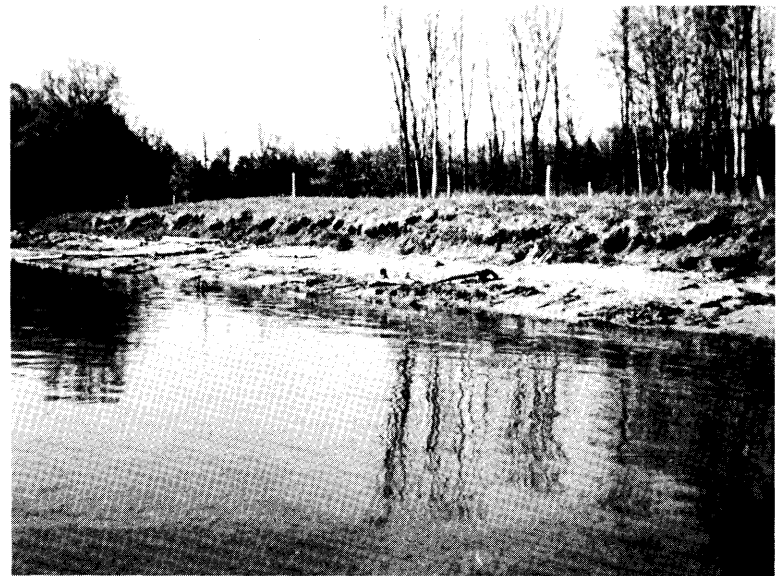
b. Newly exposed, unvegetated bank face surfaces (St. Marys reach 6c).
