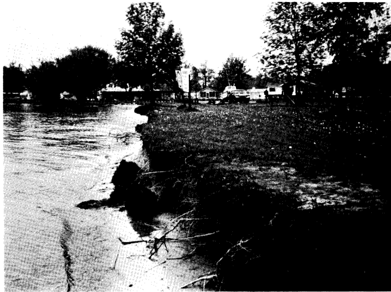
a. Slumped soil blocks (St. Clair River reach 17).
