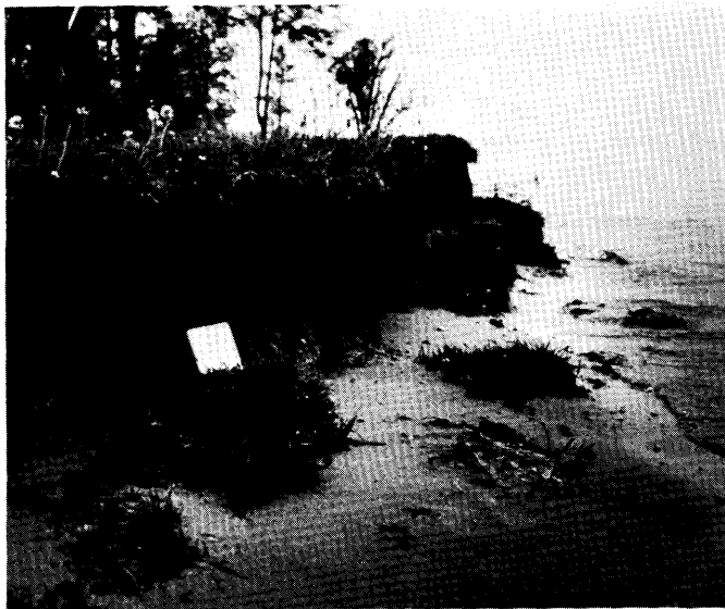
c. Removal of slumped material.
