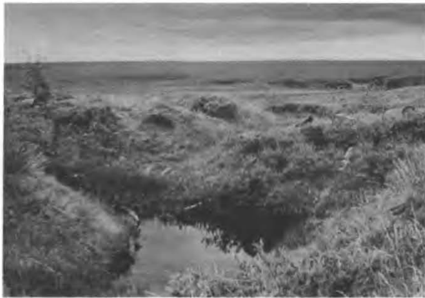
Figure 10. Former drainage ditch on north margin of site; thermal and hydraulic erosion developed channel over 3 m deep (disturbance group 4).
