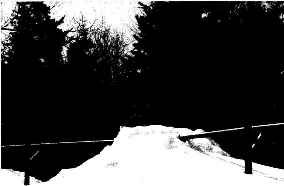
Figure 15. Sags in spray lateral 10.
