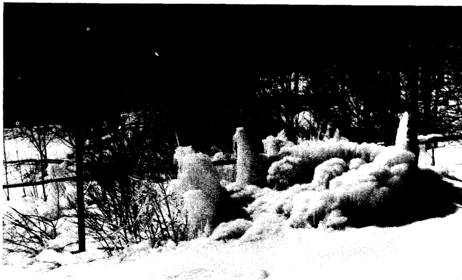
Figure 14. Snow and ice buildup near spray nozzle.
