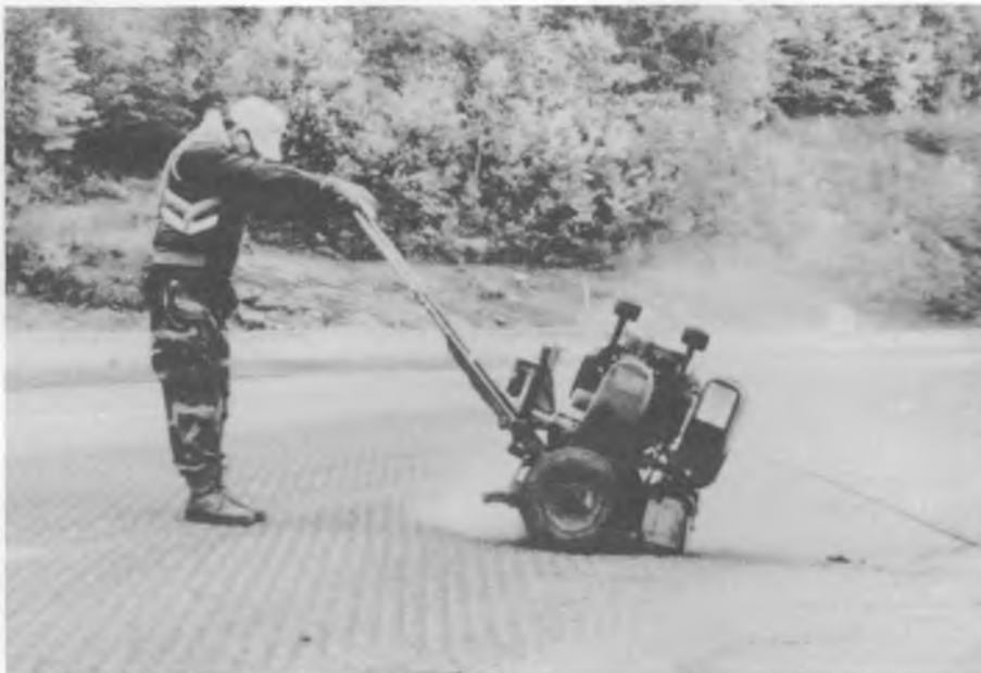
Figure 7. Routing a pavement crack prior to sealing.
