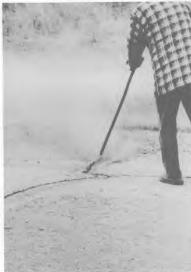
Figure 8. Crack cleaning with compressed air.
