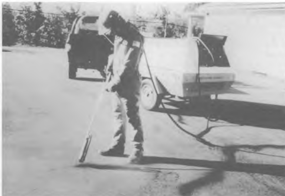
Figure 9. Hot compressed air lance.
