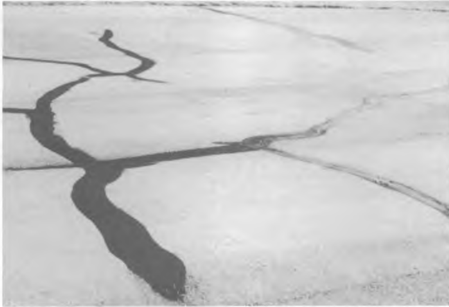
Figure 12. Sealed cracks with overbands.
