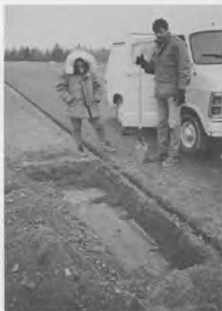
a. Trench excavation.
