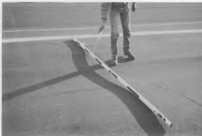
Figure 12. Differential frost heave near station 8+00. The "valley" is about 6 in. below the "ridges."
