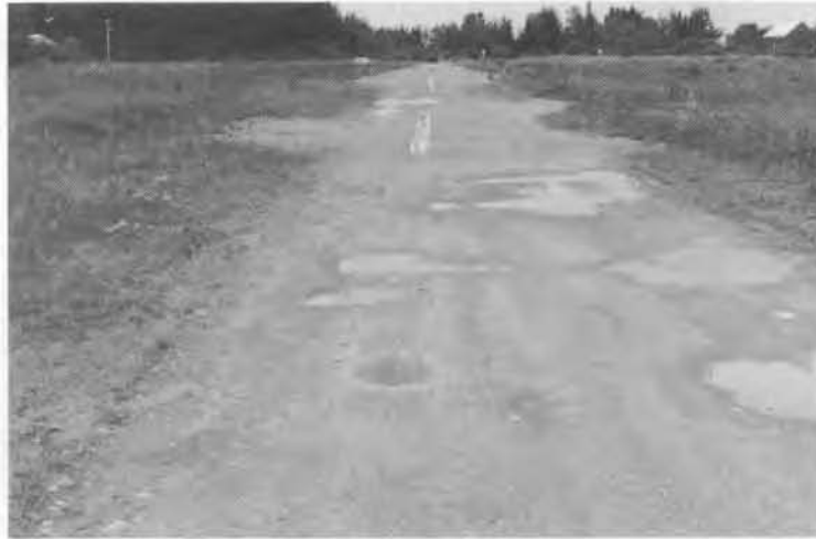
a. Looking northwest.
