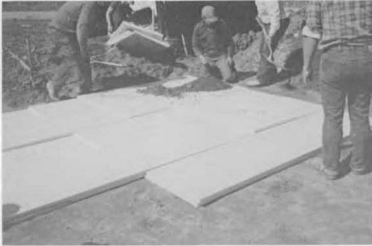
Figure 6. Placement of insulation panels at the test sections.
