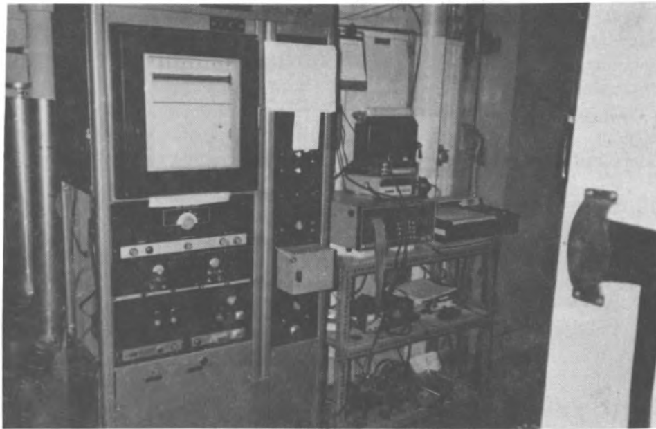
b. Operating panel and recording system.
