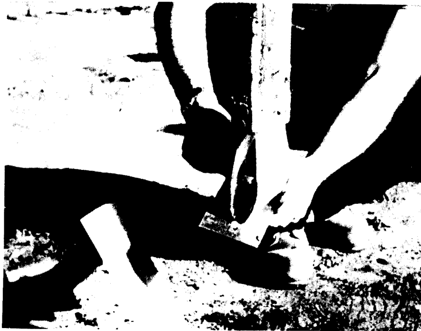
Figure 2. Vertical strip drain installation procedure
