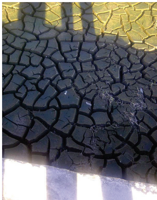
Figure 9. Sewage sludge in drying bed at American Water Operated Wastewater Treatment Plant.
