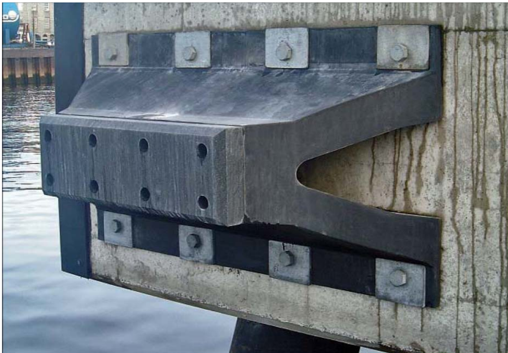
Figure 5.7 A Super Arch Delta energy absorbing system (after Trelleborg, 2007).
