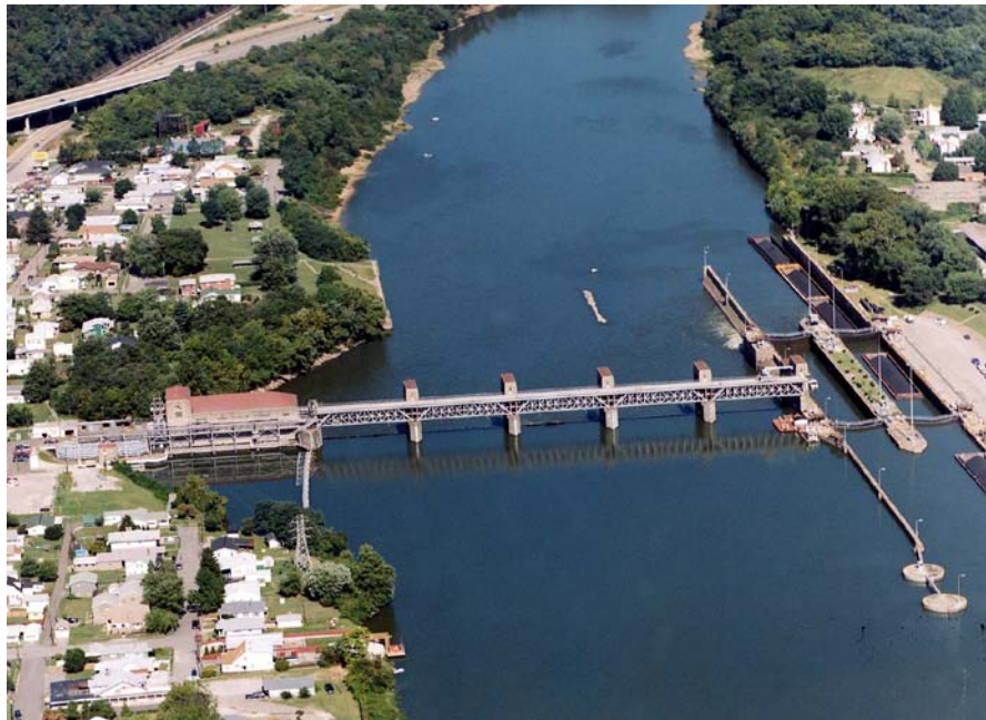
Figure 5.17 Marmet Lock and Dam with Cellular Bullnose
