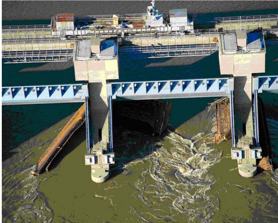
Figure 5.19. Barges blocking dam gate operations at Belleville Locks and Dam.
