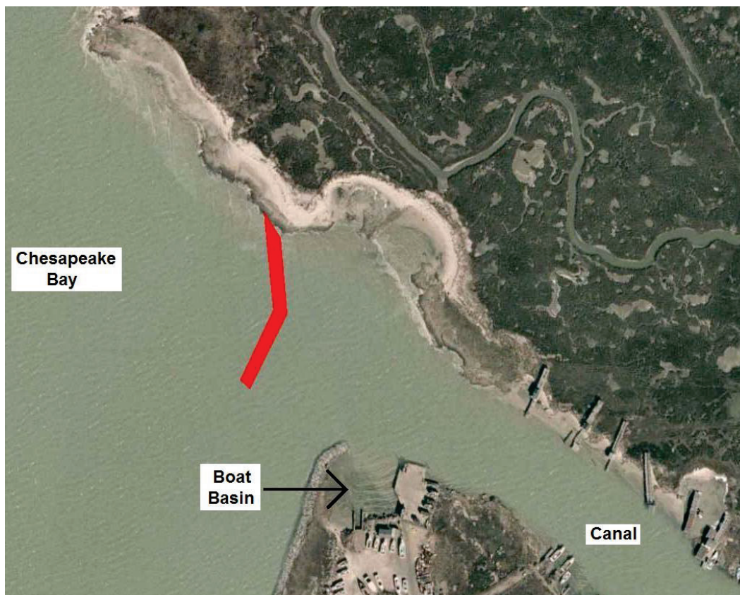
Figure 3. An example breakwater location (in red) at the western entrance of the Tangier Island boat canal.
