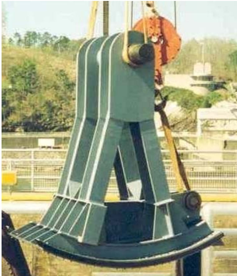
Figure 50. New (framed) reverse tainter valve, Chickamauga Lock, Tennessee River.
