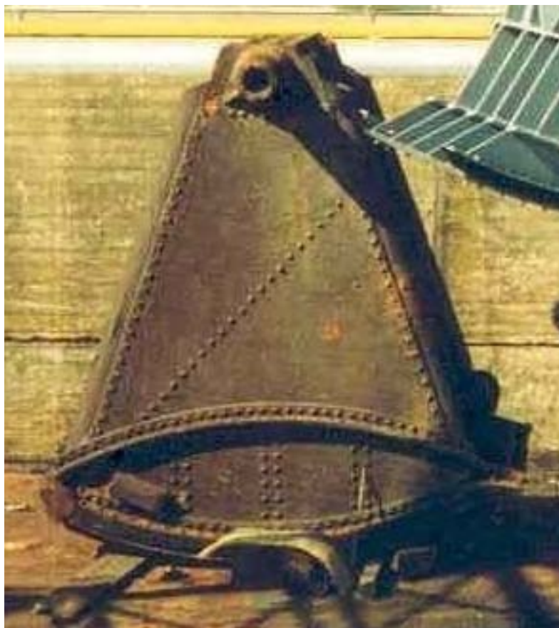
Figure 49. Old (double skin plate) reverse tainter valve, Chickamauga Lock, Tennessee River.
