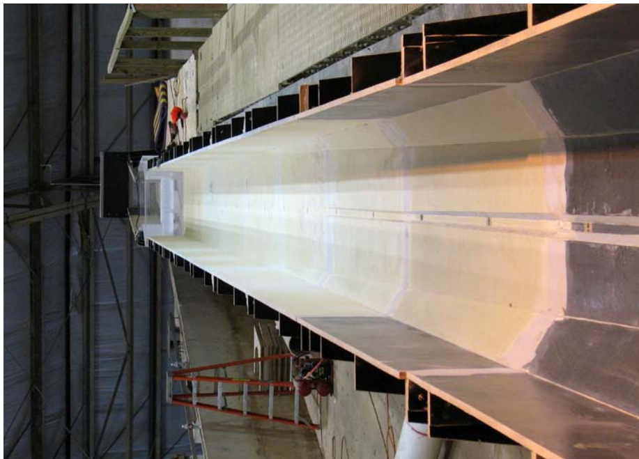
Photo 2. Channel looking downstream.
