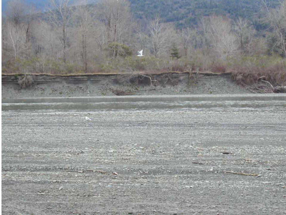
Figure C58. XC27 (right bank) - Looking at erosion of left (gravel) bank
