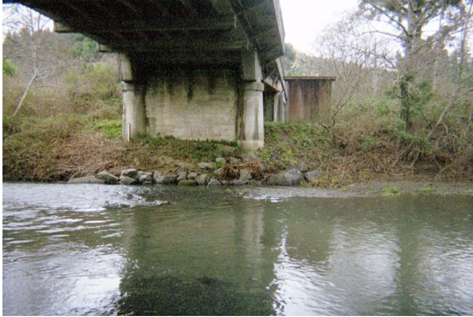
Figure D6. North Fork Mad River -1928 Blue Lake (Korbel) bridge abutment
