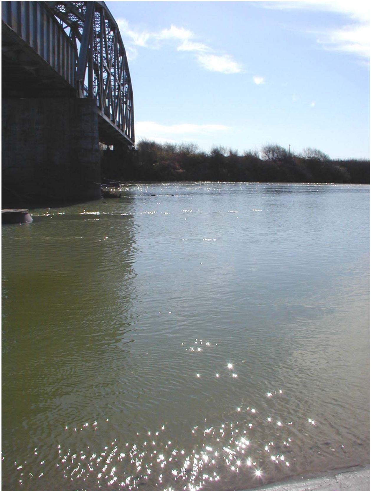
Figure C4. XC3 (right bank) – Looking under old railroad bridge
