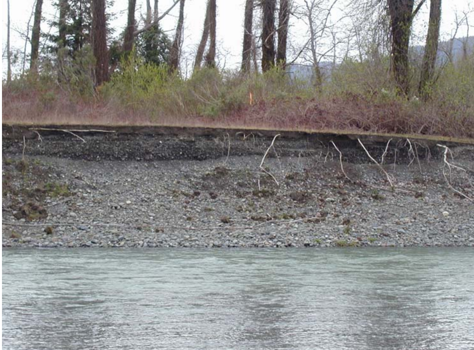
Figure C62. XC28 (right bank) - Looking at erosion of left (gravel) bank
