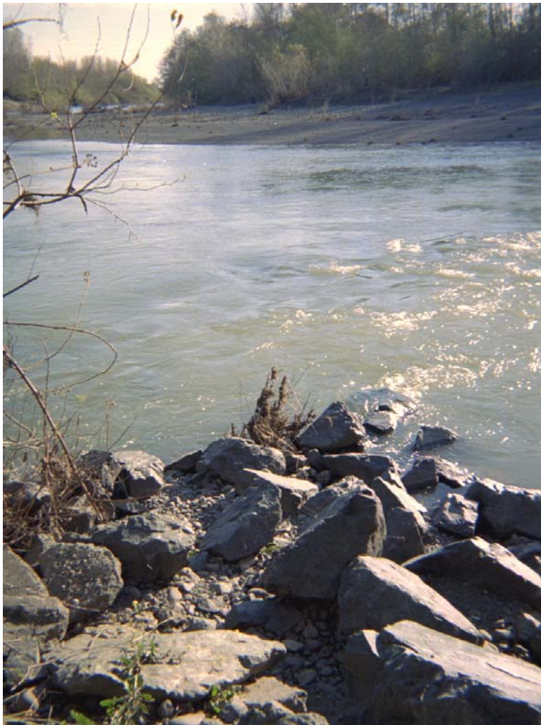
Figure C18. XC12 (right bank) – Looking from fill and riprap
