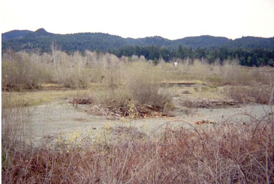
Figure C57. XC27 (right bank) – Standing on levee at cross section end point
