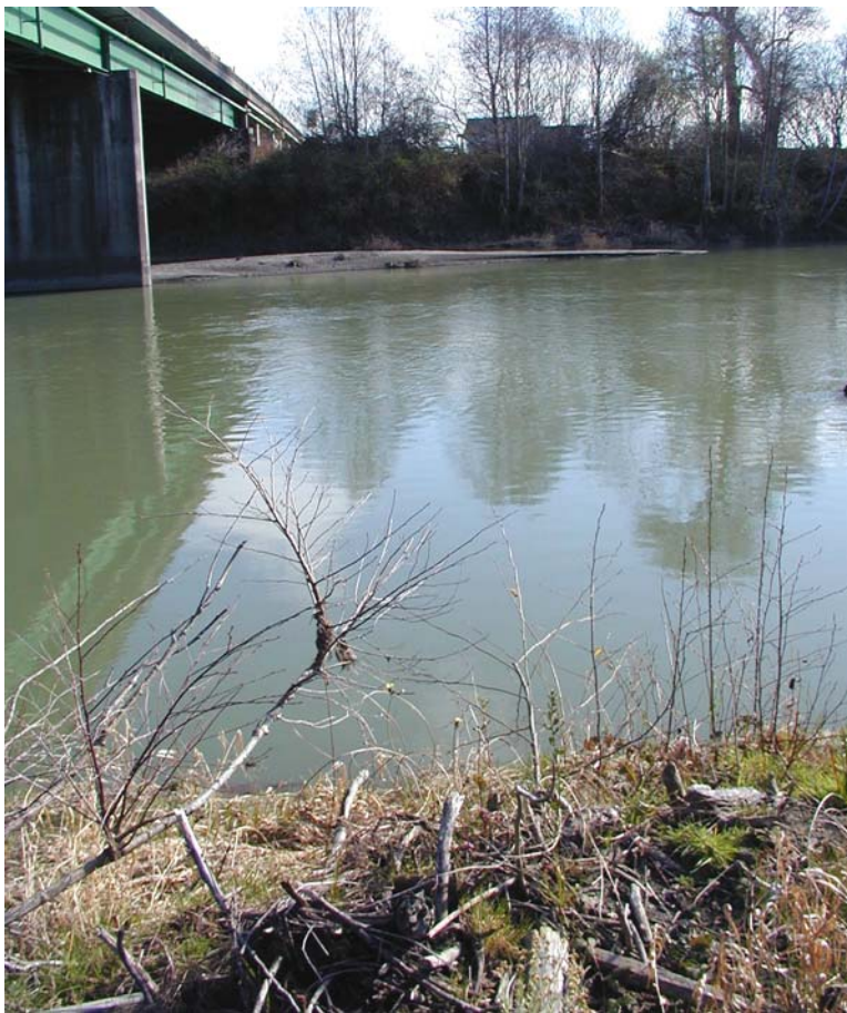
Figure C12. XC9 (right bank) – Highway 101 bridge
