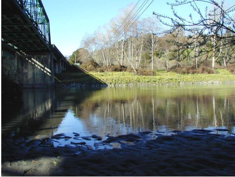
Figure C13. XC10 (left bank) – Highway 101 bridge
