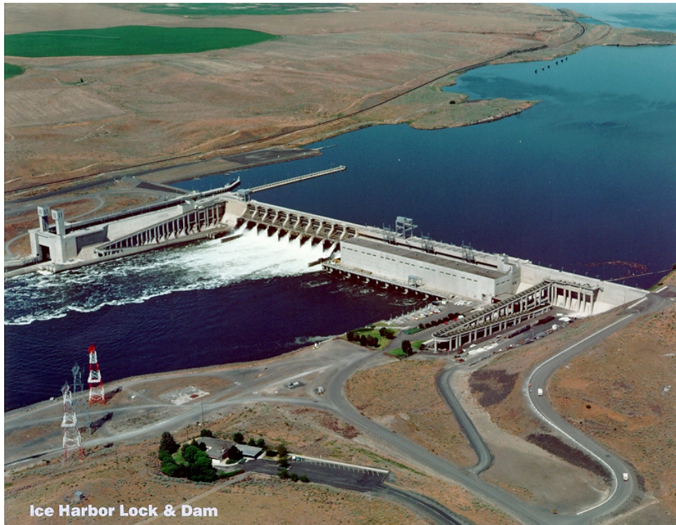
Figure 3. Ice Harbor Lock and Dam (powerhouse, spillway, and navigation lock)
