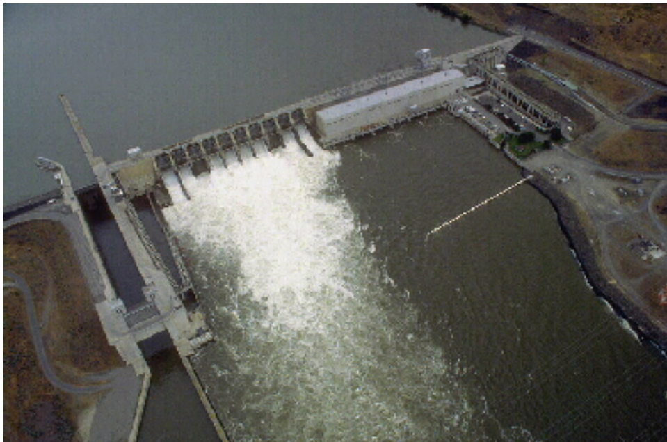
Figure 2. Ice Harbor Lock and Dam (forebay at top of photo)
