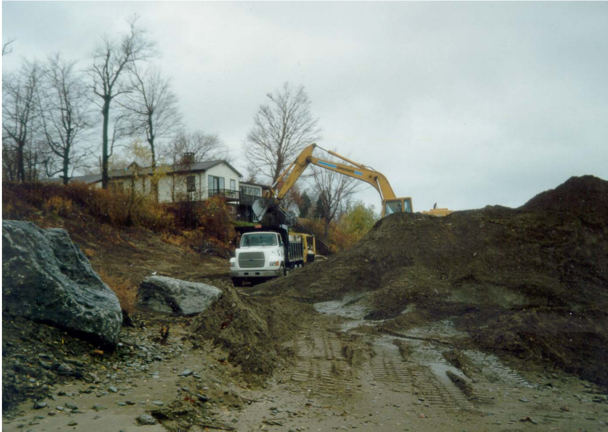
Figure 25. West fillet sediment being loaded into dump trucks, 17 November 1998
