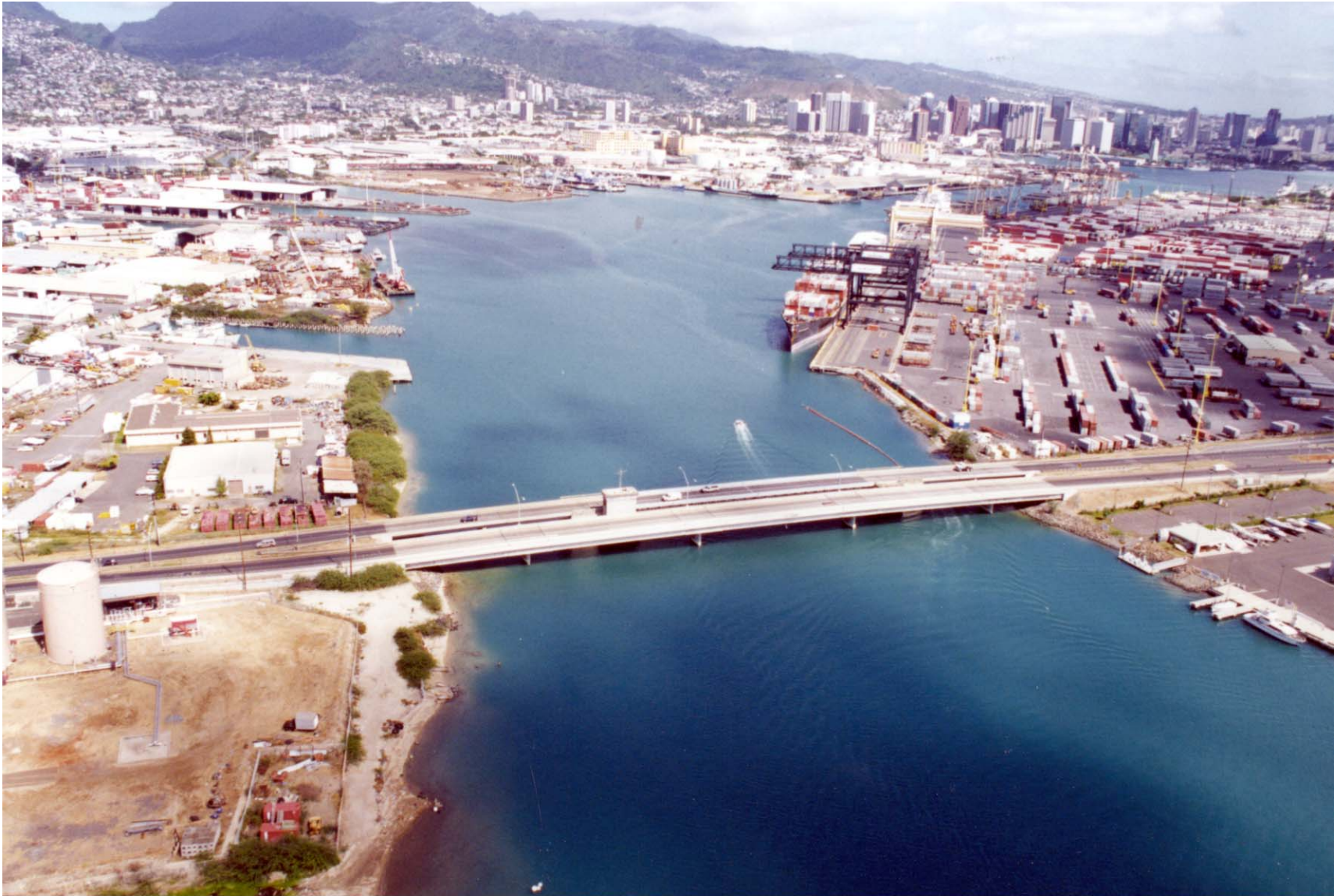
Figure 2. Sand Island Bridge
