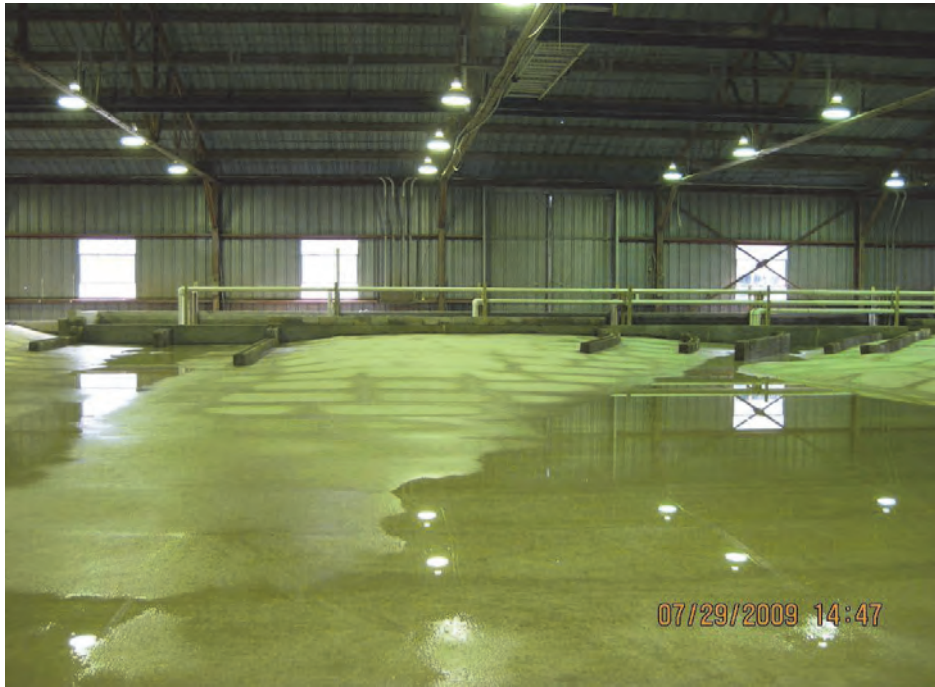
Figure 17. Approach walls used to guide flow from Algiers and Harvey Canals.
