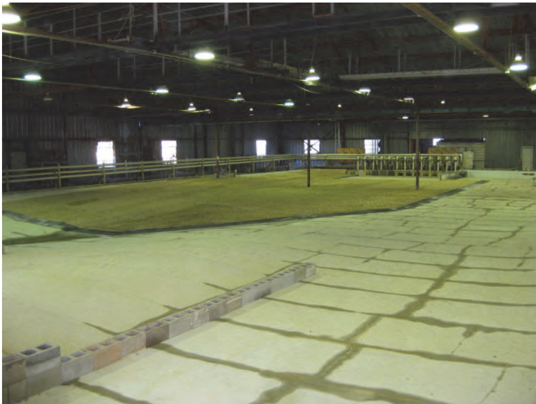
Figure 19. View of revised approach channel looking downstream.
