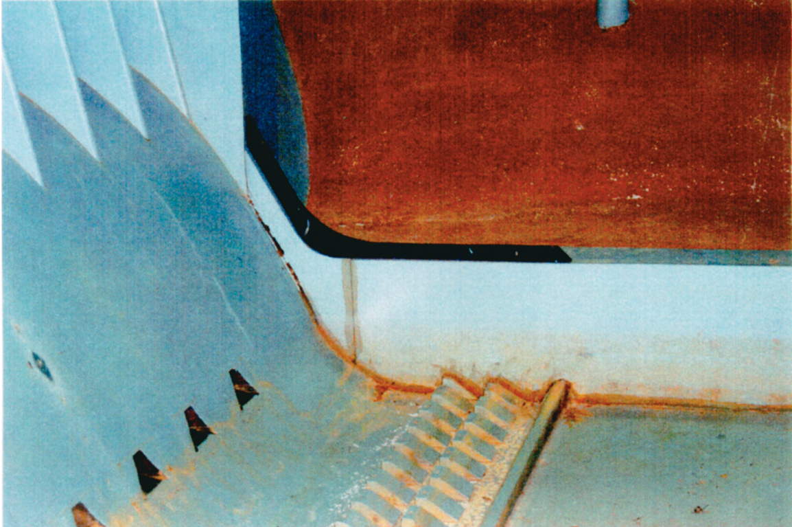
Photo 3. Final west training wall extension
