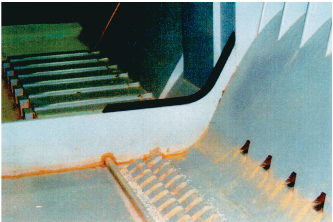
Photo 4. Final east training wall extension
