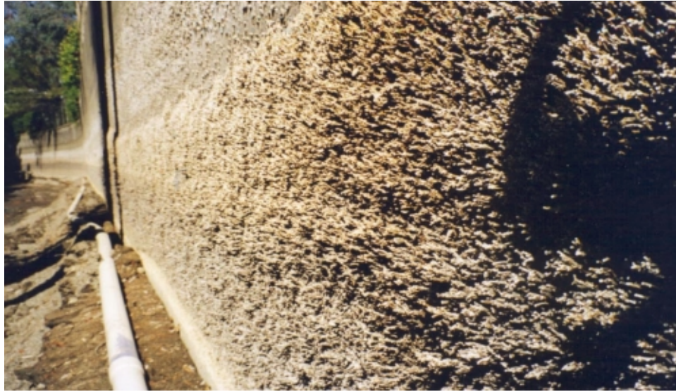
Figure 4. Tube worm and barnacle growth Station 323+00
