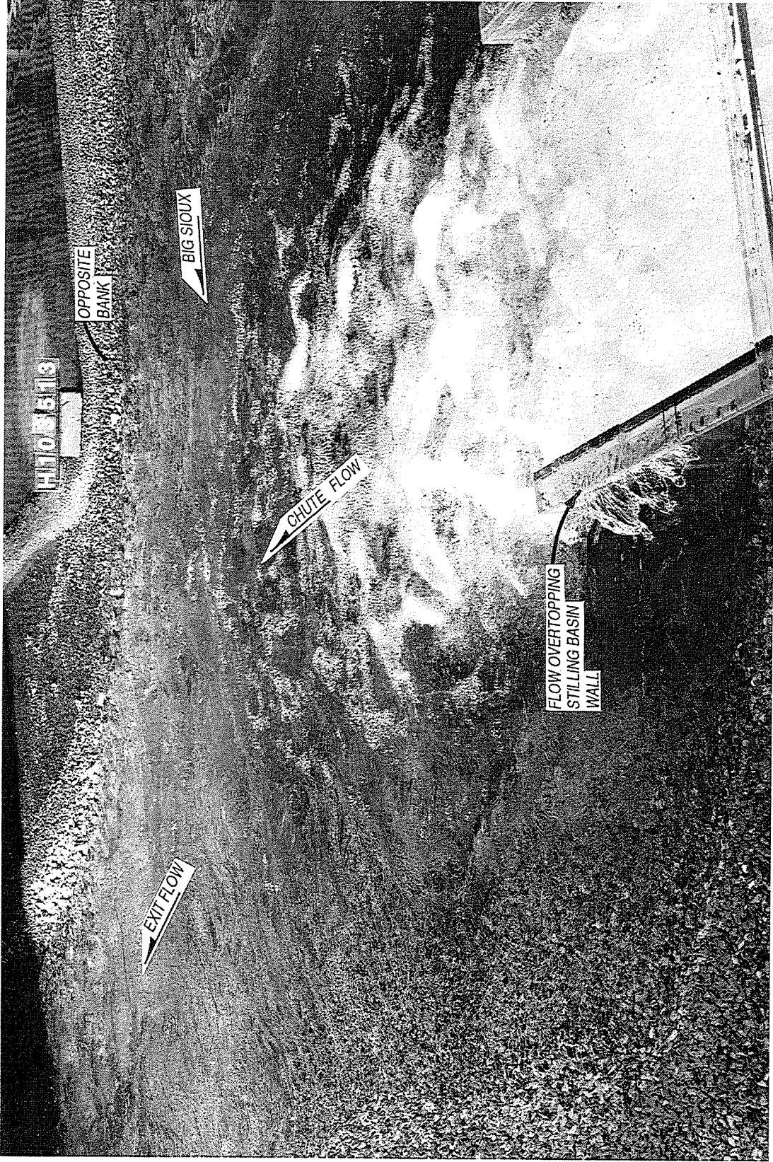
Photo 11. Type 2 stilling basin; 1969 flood; Q_c 812 cu m/sec (29,000 cfs); Q_r 316 cu m/sec (11,300 cfs); tailwater el 1324.5
