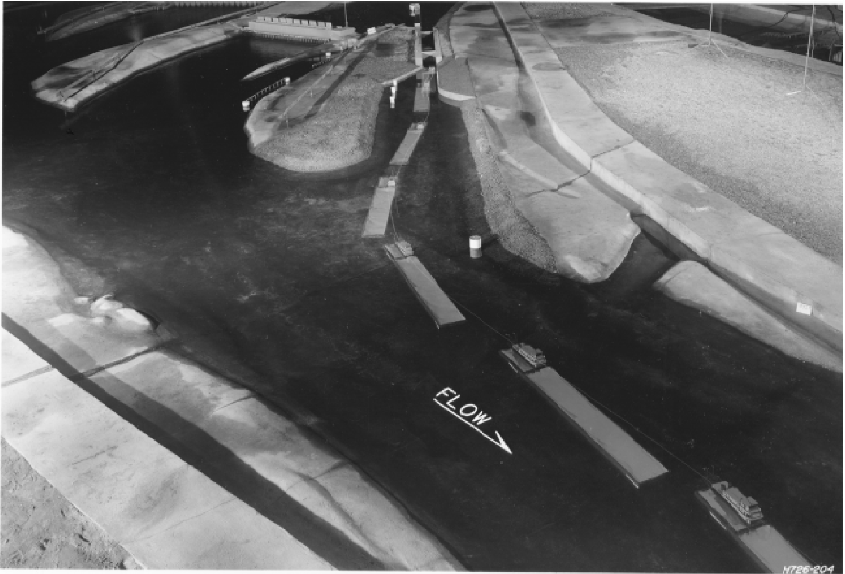
Photo 11. Plan F, looking upstream, 335,000 cfs total riverflow, showing path of downbound tow leaving new lock
