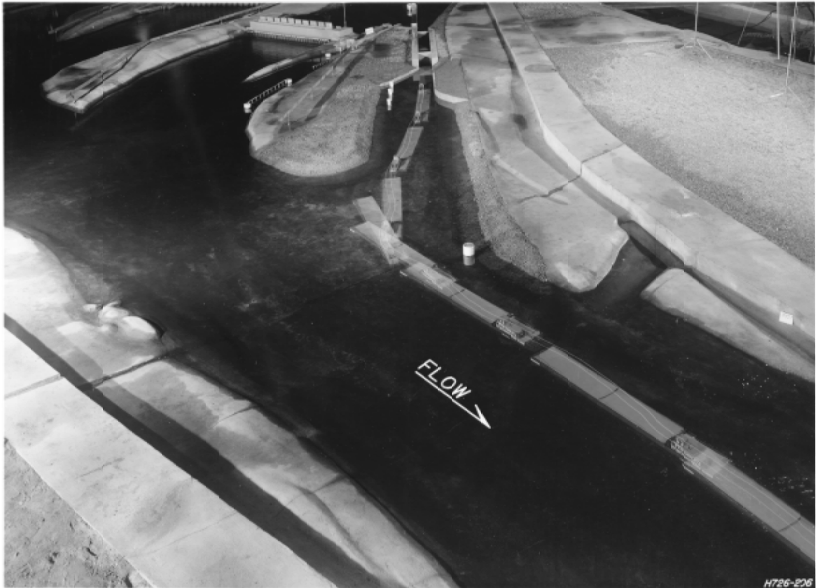
Photo 12. Plan F, looking upstream, 335,000 cfs total riverflow, showing path of upbound tow approaching the new lock
