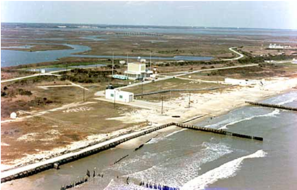
Figure 2-11. Condition of groins and seawall in 1983.
