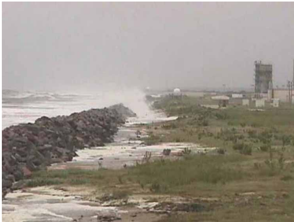
Figure 2-15. Rock seawall during Hurricane Dennis, September 1999.
