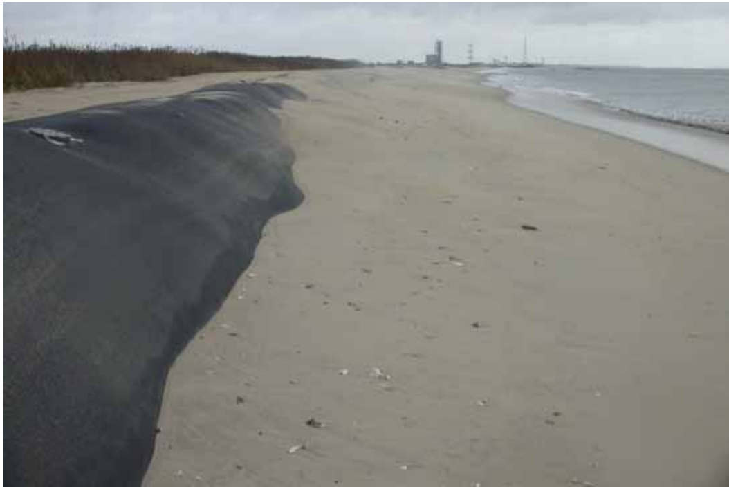
Figure 3-7. Looking north from southern portion of geotextile tube.
