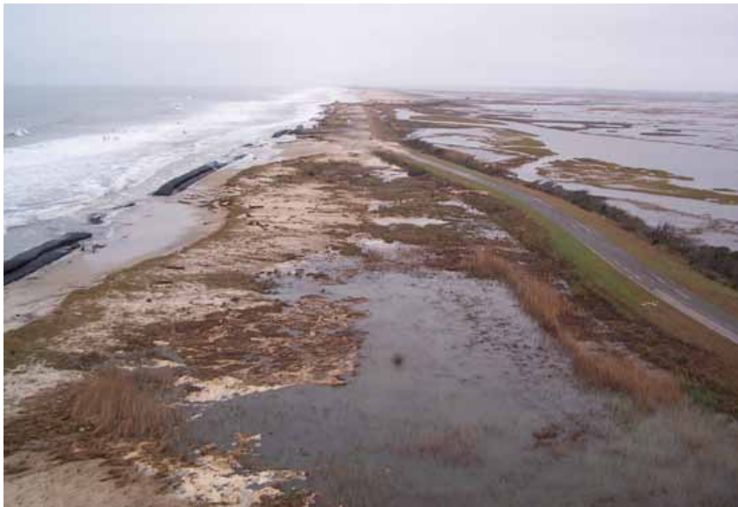
Figure 2-17. Damage to the south end of Wallops Island caused by the November 2009 nor'easter.
