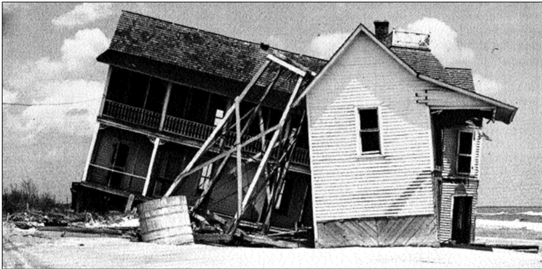
Figure 2-4. Wallops Island north end erosion damage, May 1949.
