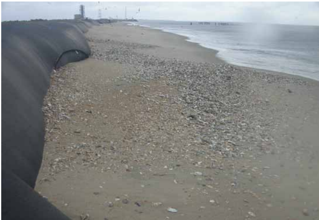
Figure 3-8. Near the middle of the geotextile tube section, looking north.
