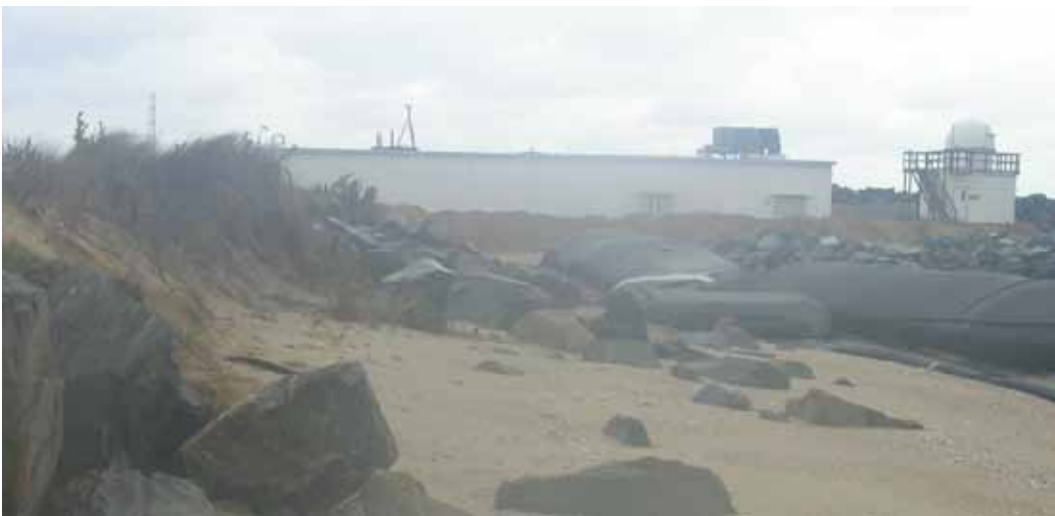
Figure 3-10. Short geotextile tube behind the north end of main tube.
