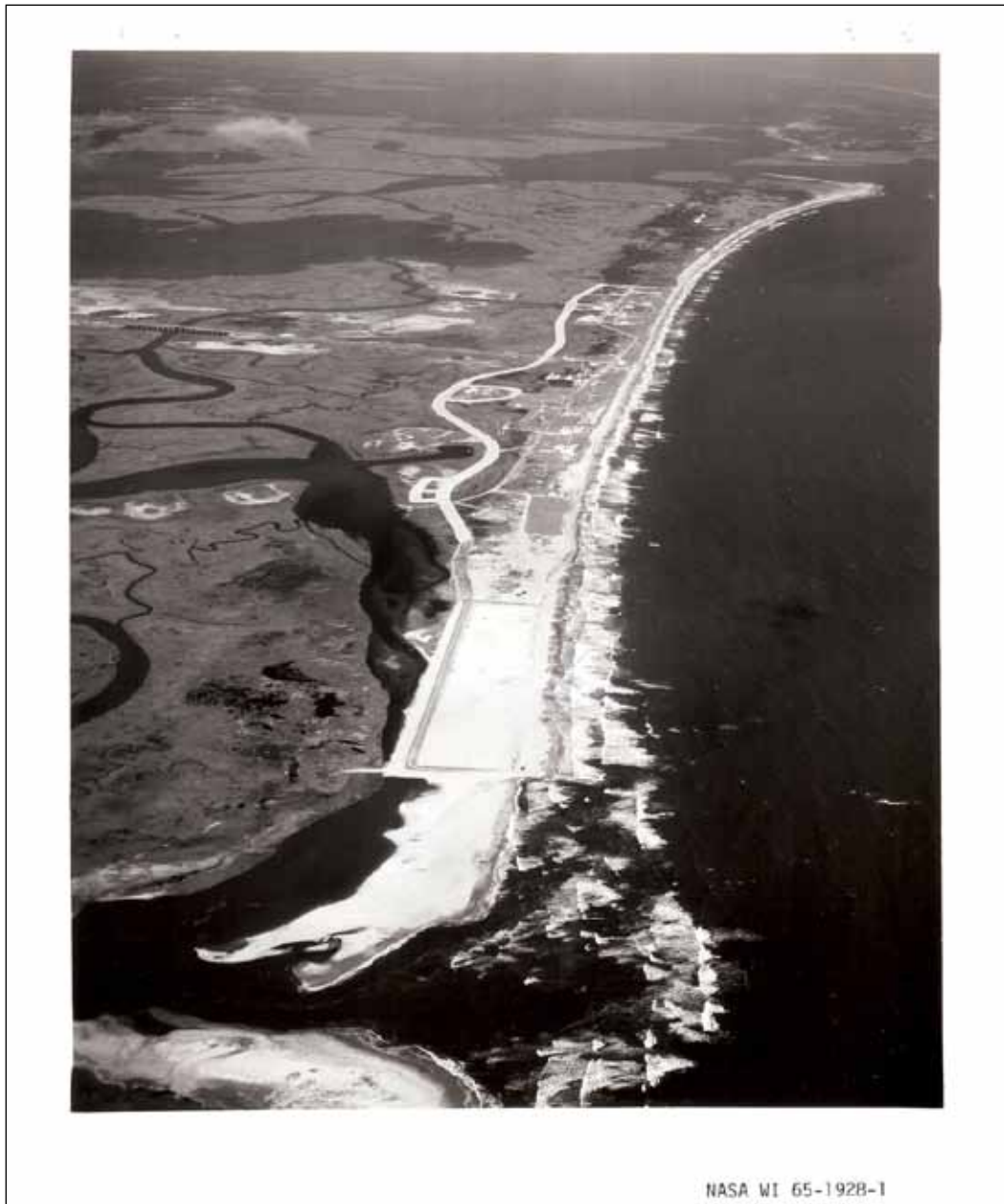
Figure 2-8. Mechanically filled section of the south end of Wallops Island following an Ash Wednesday Storm breach.
