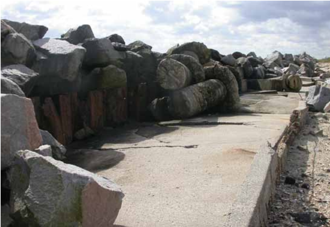
Figure 3-15. Remnants of concrete apron with steel sheet pile wall.
