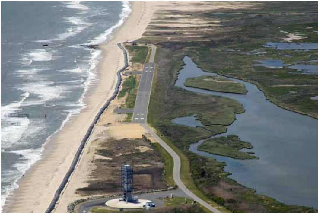
Figure 2-16. 2007 oblique aerial photo looking south from near the south end of Wallops Island, Va. From bottom to top the shoreline shows the geotextile tube and the overwash area that was previously Assawoman Inlet.
