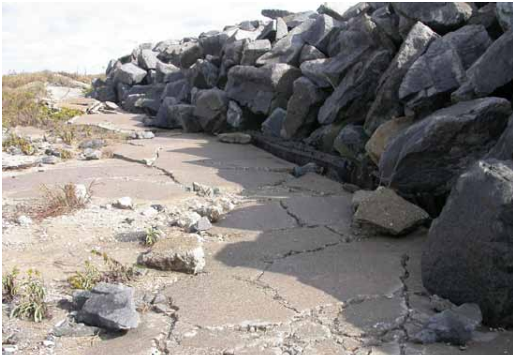
Figure 3-14. Remnants of concrete apron and timber pile wall.
