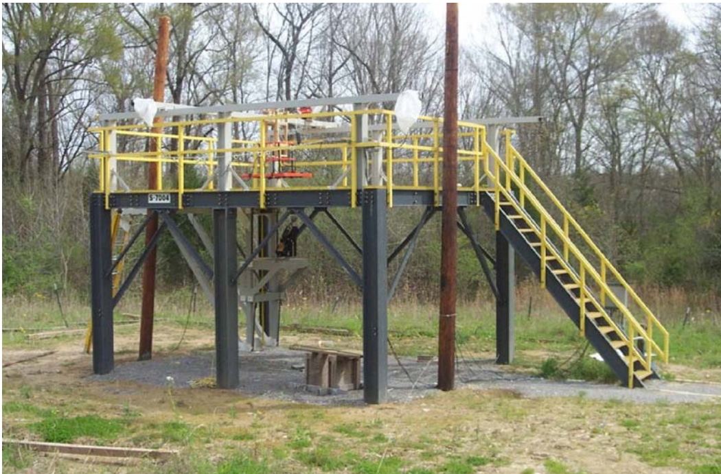
Figure 1. View of the ERDC test stand from the north.
