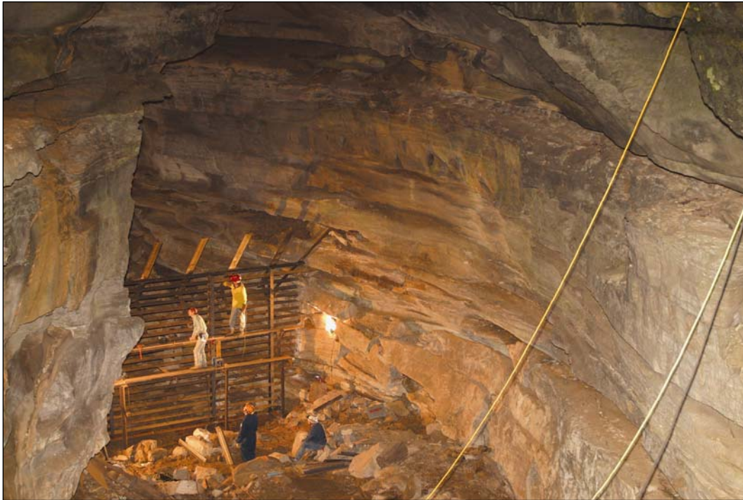
Figure 8. Hubbards Cave gate replacement in May 2006 (photo courtesy of J. Kennedy, BCI).
