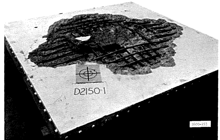
d. Slab with column removed.
