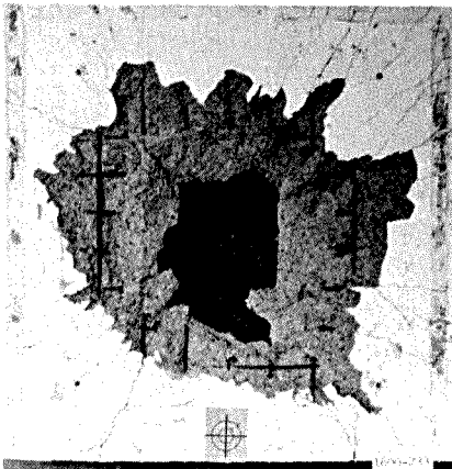
c. Column removed, cracks marked.
