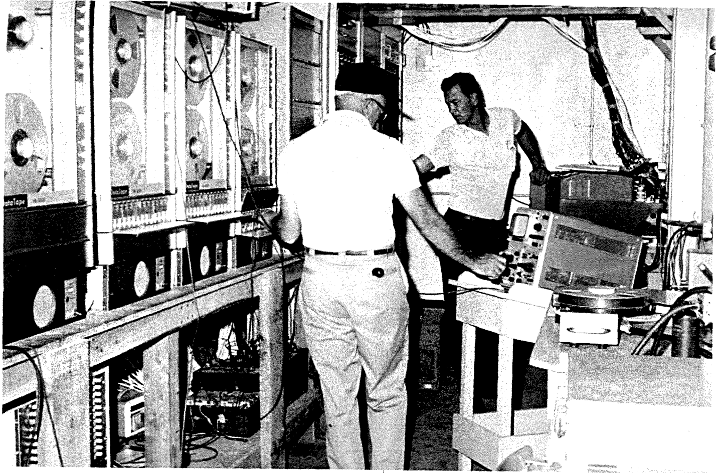
Figure 2.4 Interior of instrument bunker.
