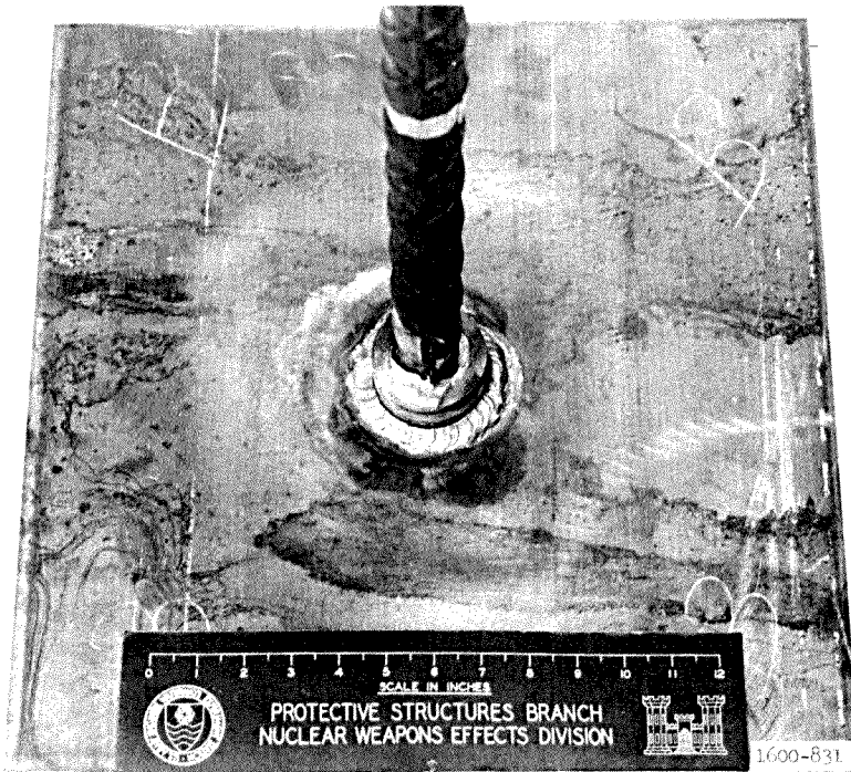
Figure 3.16 Separation of joint from Cadweld sleeve, Test 13 (Cadweld-spliced bar).
