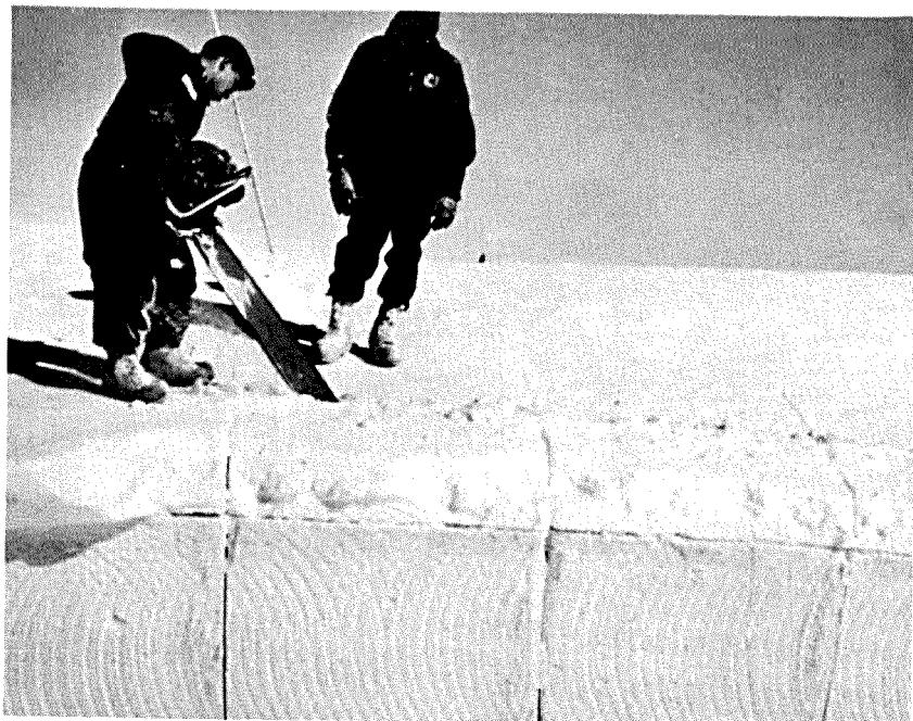
Figure 2.19 Cutting blocks from a pad of processed snow with a gasoline-powered chain saw.
