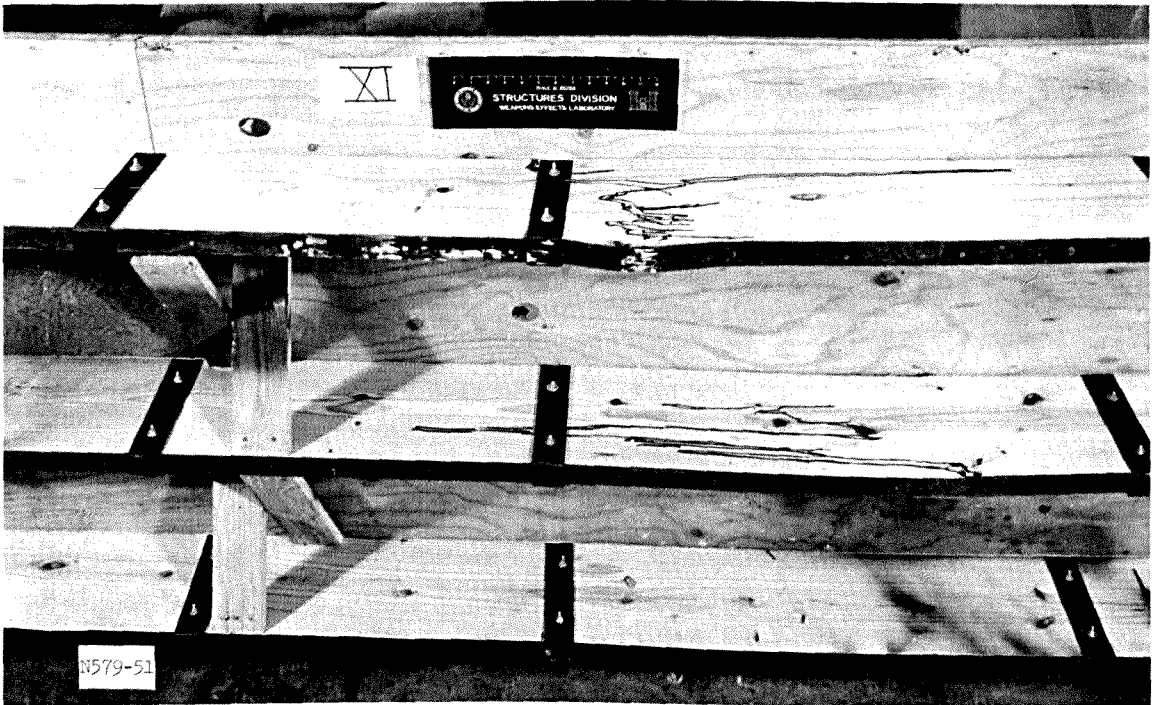
b. Close-up of joist failures.
