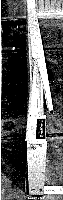
a. Joist failure (note plywood nail pullout).
