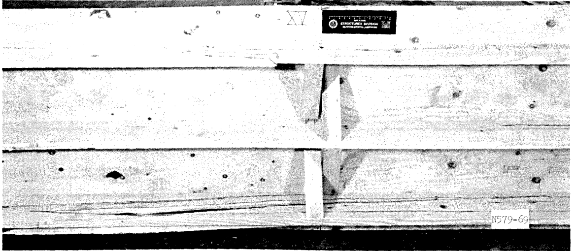
b. Close-up of joist failures.
