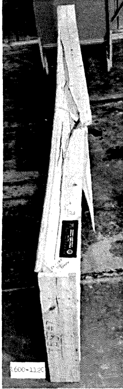
a. Joist failure.
