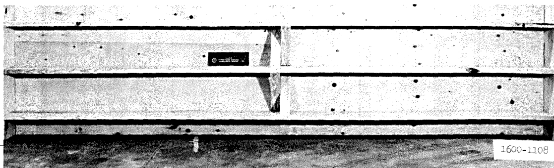
b. Bottom view of unreinforced test specimen (I).
