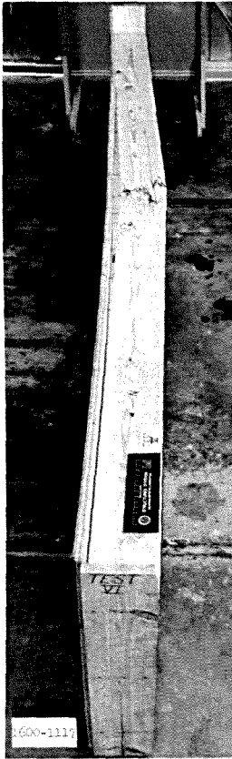
a. Joist failure (note plywood nail pullout).
