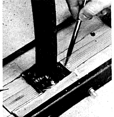
RIB SHOWN IN PLACE POSTSHOT 5
