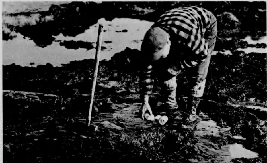
(c) Drilling a hole for a dynamite charge
