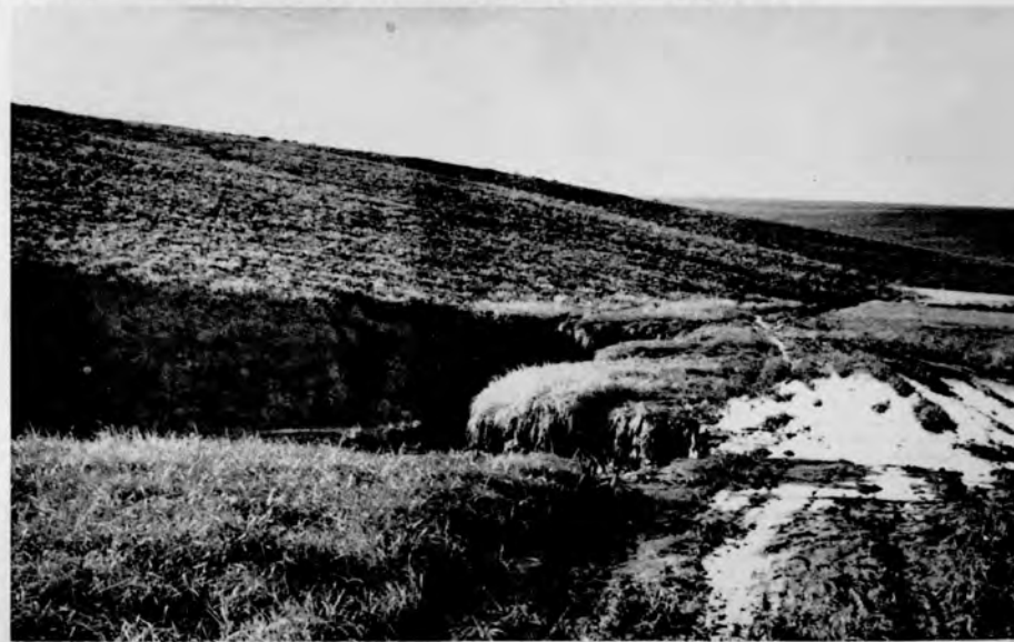
(d) Gullying along the shoulder, Umiat
