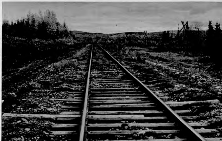
(b) Fill settlement in frozen silt, near Goldstream
