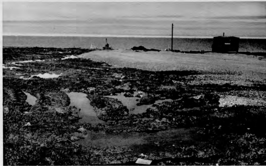
(b) Placing a gravel fill on thawing peat and silt
