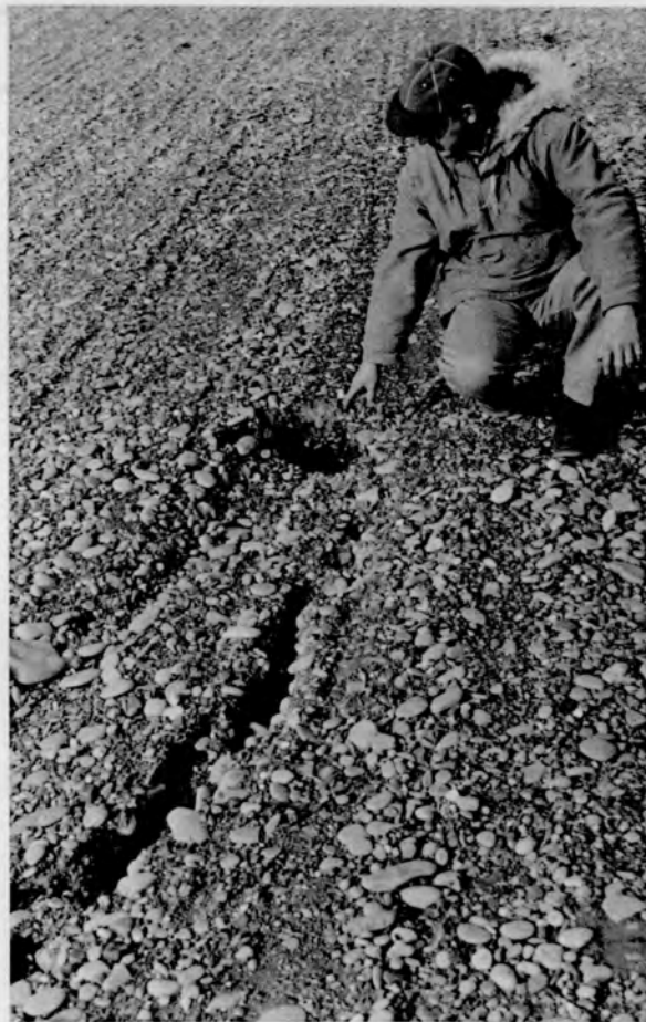
(b) Crack in a gravel surface
