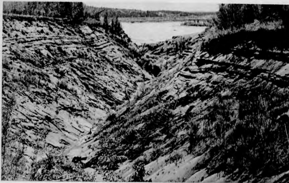
(a) Unchecked highway culvert effluent
