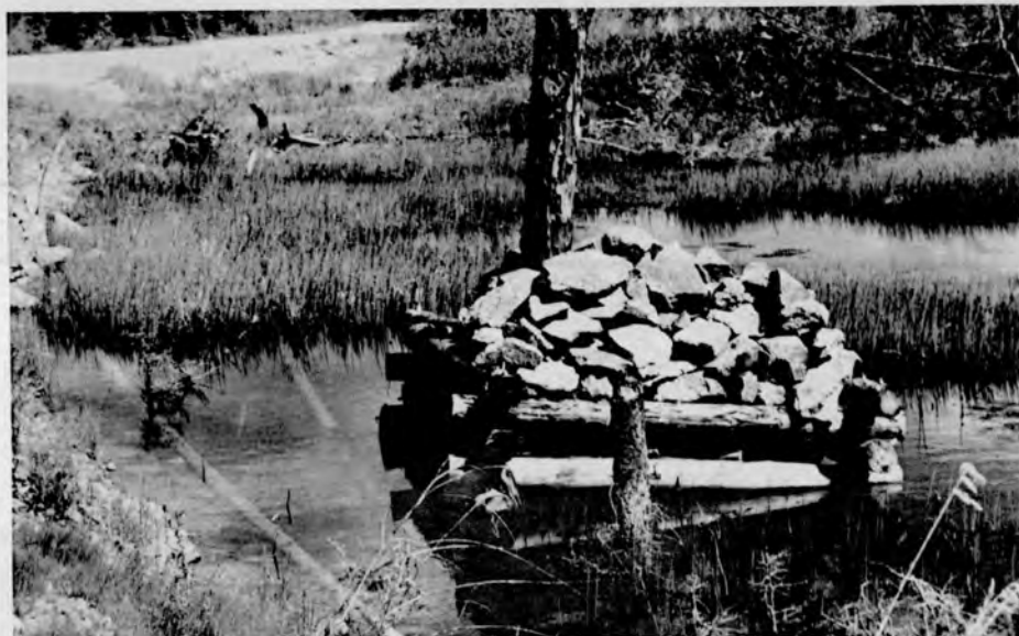
(b) Telephone pole construction in permafrost areas
