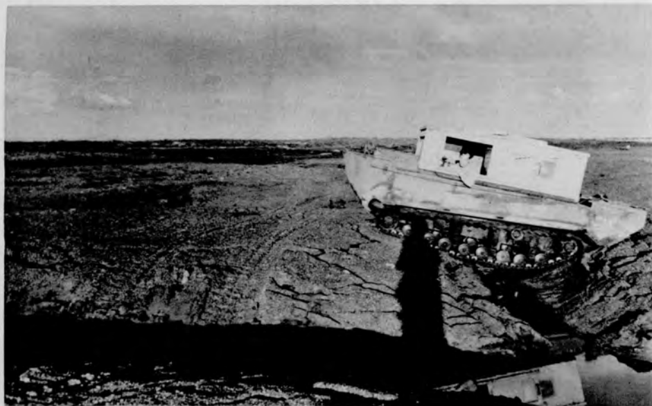
(c) Thaw cracks in the winter runway
