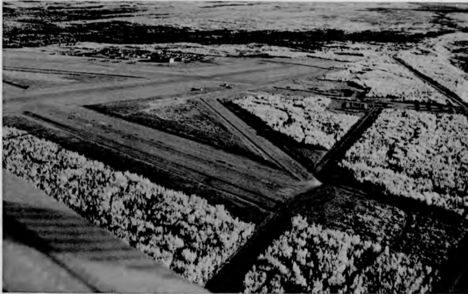
(a) Runways on gravel terrace
