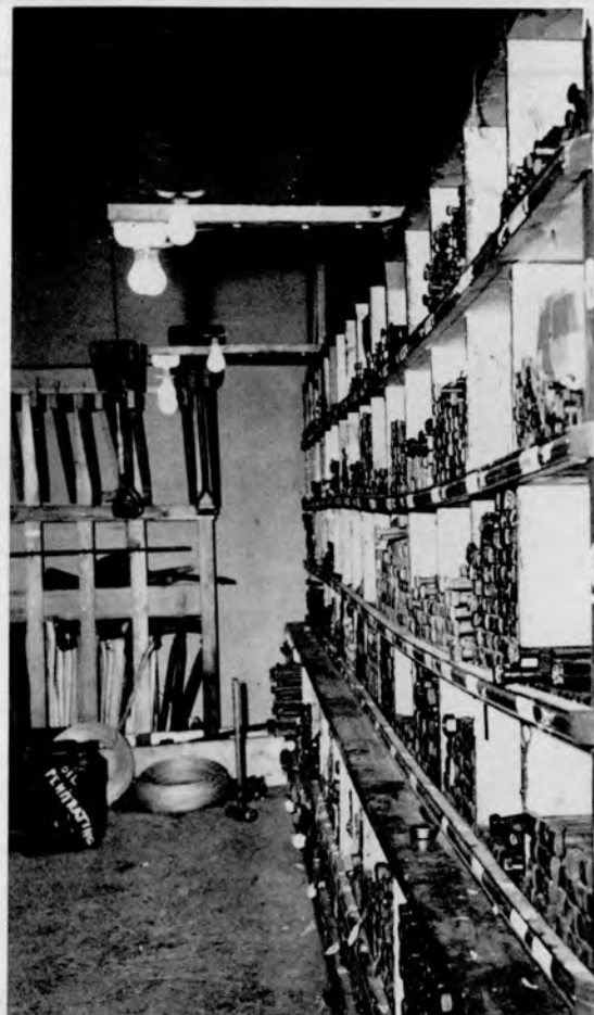
(b) Floor settlement in a warehouse
