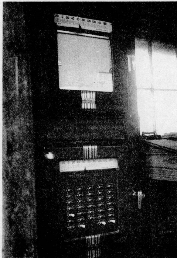
FIG. 2 VIEW OF TEMPERATURE MEASURING POTENTIOMETERS.
