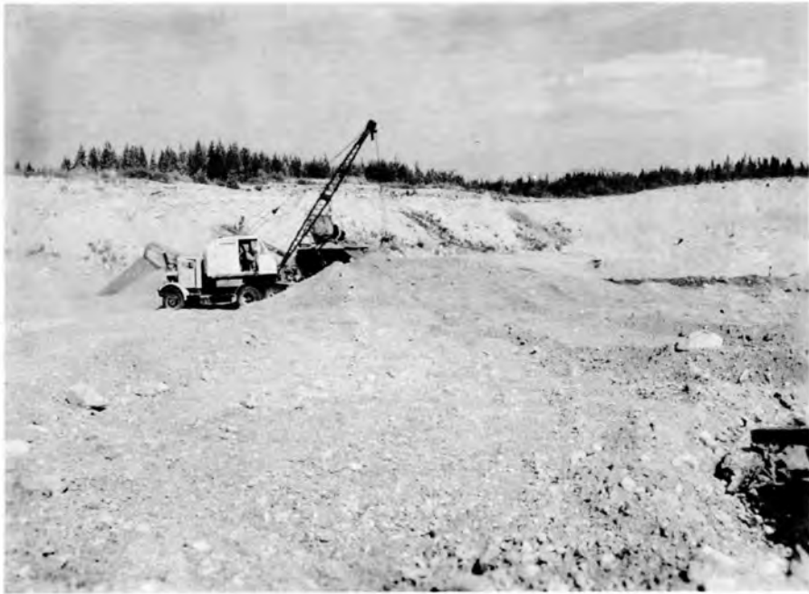
Fig. 15. Gravel pit adjacent to the Alaska Highway near Whitehorse.
