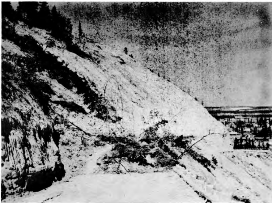
Fig. 9. A landslide caused by the silts becoming saturated and flowing during wet weather.
