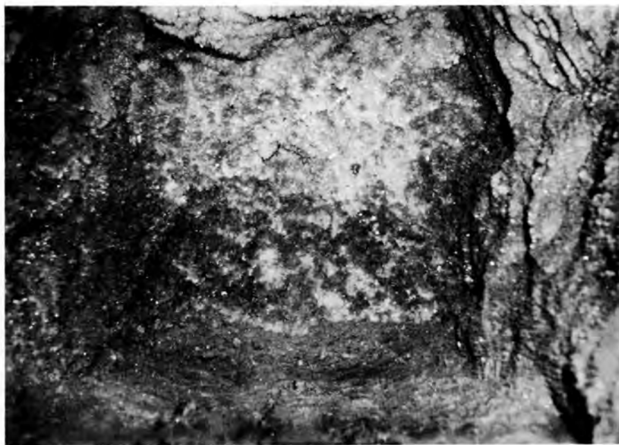
Fig. 97. Ice crystals formed in unventilated tunnel at 115-ft level of Giant Gold Mine No. 2 at Yellowknife.
