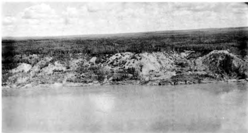
c. Landslide in drift deposits near Old Fort Point. Notice flat to gently rolling terrain.
