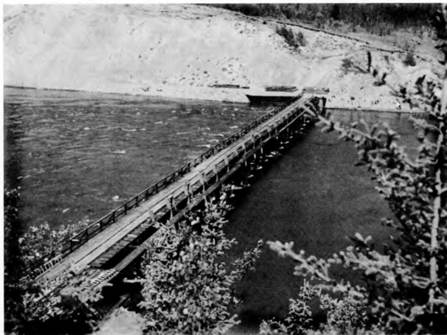
Fig. 18. The Yukon Navigation Dam. Notice the deep sands on the east side of the river.
