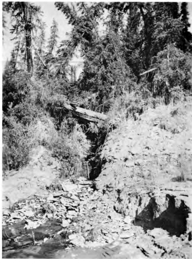
b. Figs. 52a and 53a were taken at site which is about 100 ft from this gully. Notice alluvial materials overlying shales.
