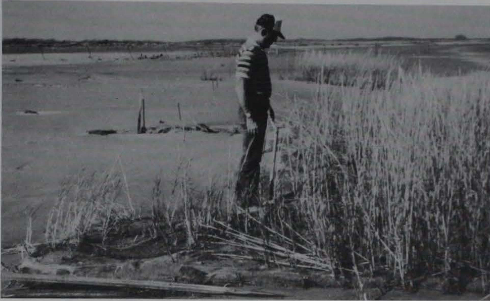
Figure 5. Single stems of smooth cordgrass to be planted in slits cut in paratex erosion control mat
