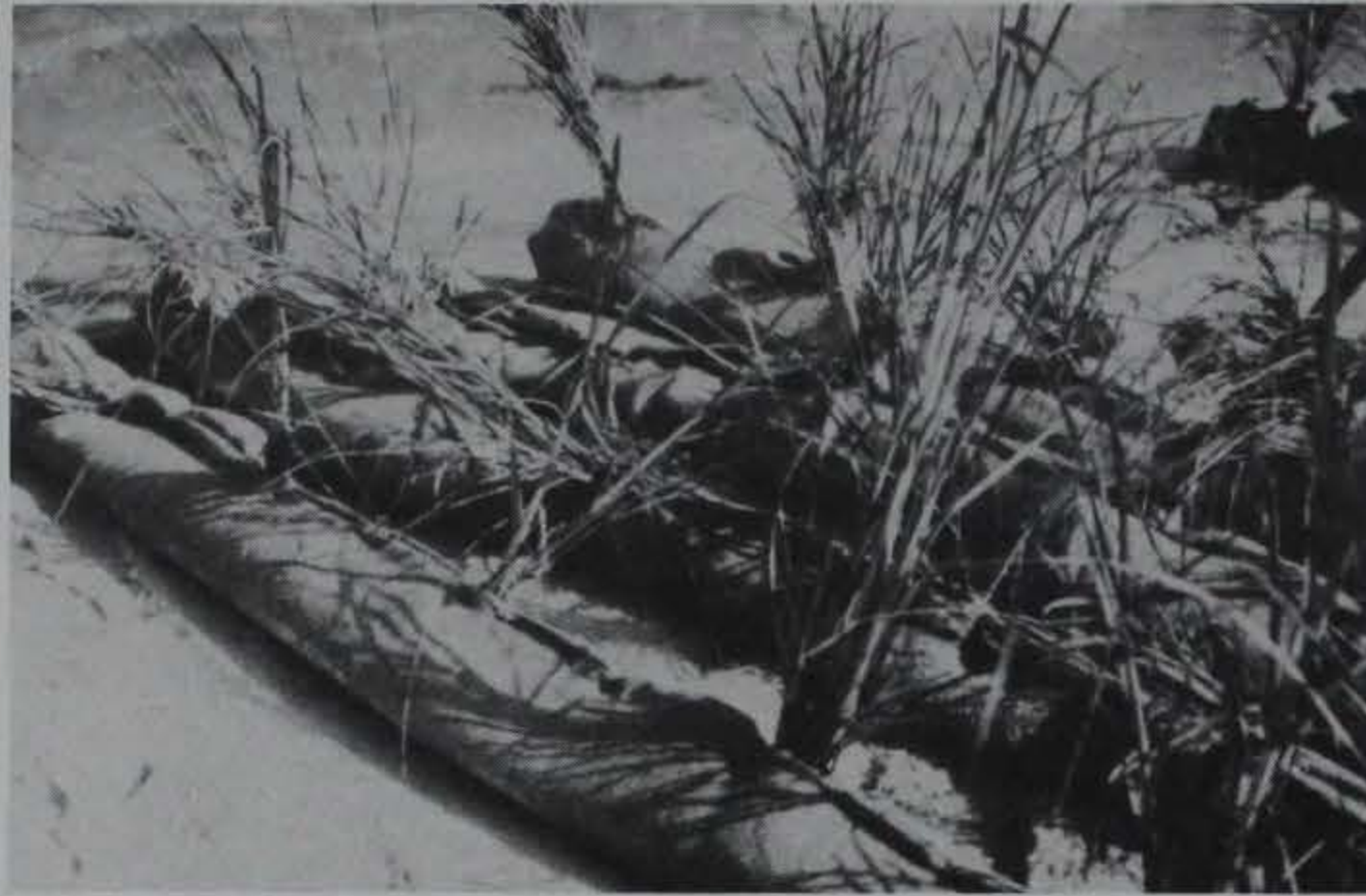
Figure 6. Plant rolls waiting to be placed along the dredged material shoreline at Gaillard Island, Alabama
