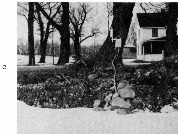
Figure 47. Photographs of the temperature recording installation on the north shore of Wamplers Lake, Winter of 1952-53. a. anemometer and recorder locations. b. Recorder house. c. Junction box, air thermometer housing and shore end of cables.
