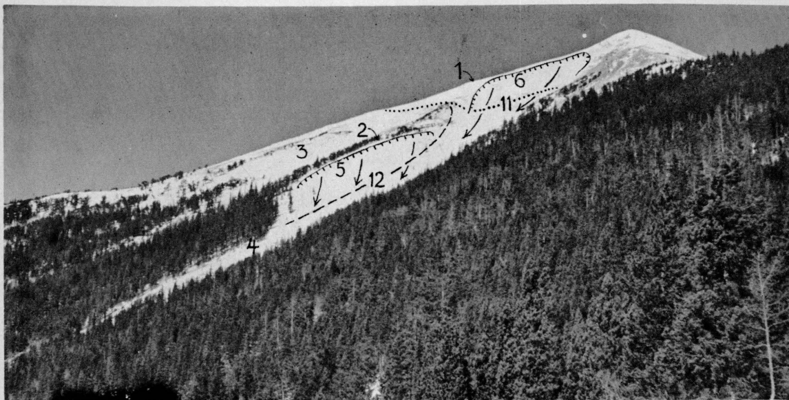
Figure 6. Upper part of Stanley Park slide, Berthoud Pass. For explanation of numbers, see text. (Photograph by E. LaChapelle.)
