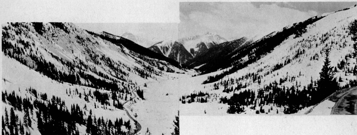
Figure 16. Highway Silverton-Red Mountain Pass, Colorado. View from the road of Bullion King (to south). An 8000-ft stretch of highway gets many small slides from the east and one big slide from the west. A compact timber on both sides of the valley would be the best protection. But one cannot yet see if trees would grow everywhere. (Photograph by A. Fuchs.)
