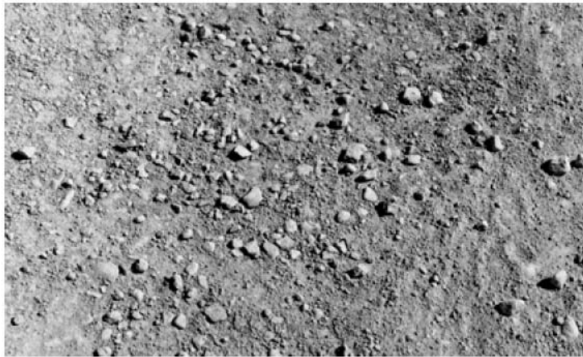
Loose Aggregate, Amber Severity
