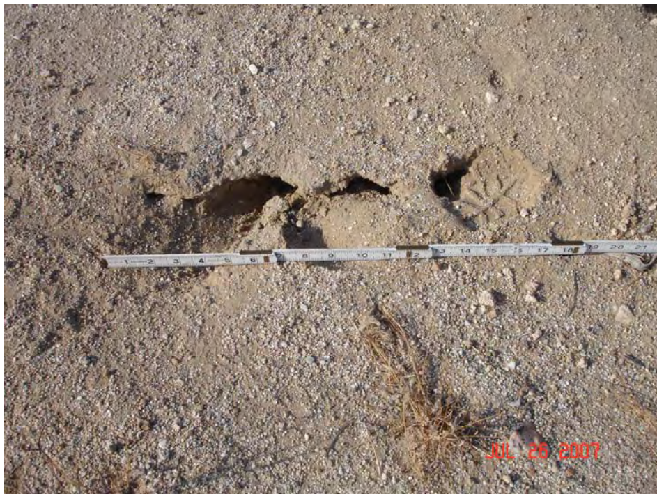
b. One of several animal holes observed on the PCI-RAS, showing a depression after a footstep.
