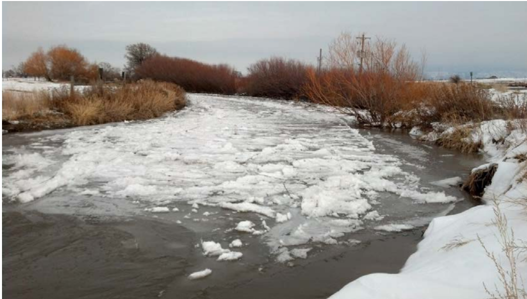
Figure 36. Ice cover in place upstream of the check dam (looking upstream).
