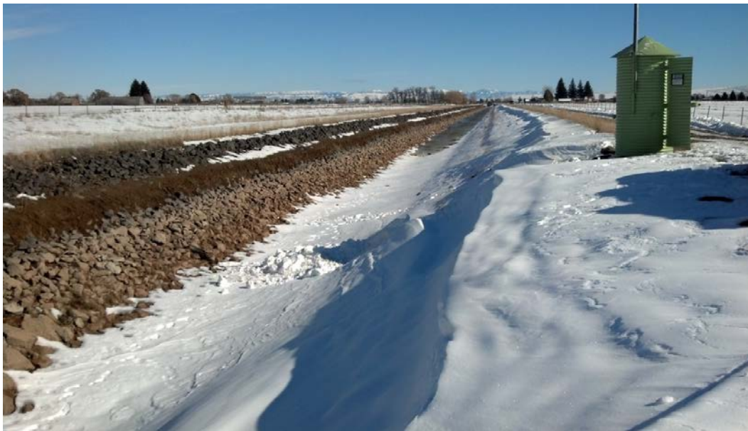
Figure 27. Looking upstream from the mouth of the Floodway Channel during release.
