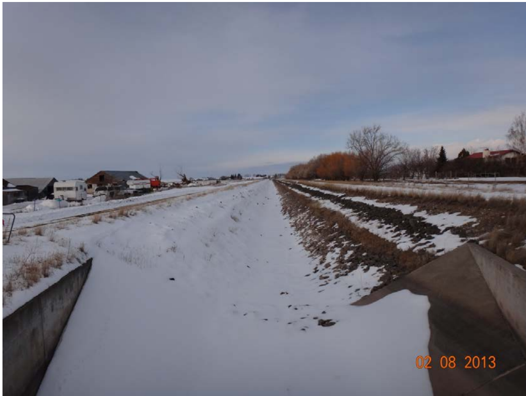
Figure 25. Looking downstream from the 5 th St. Bridge prior to release.
