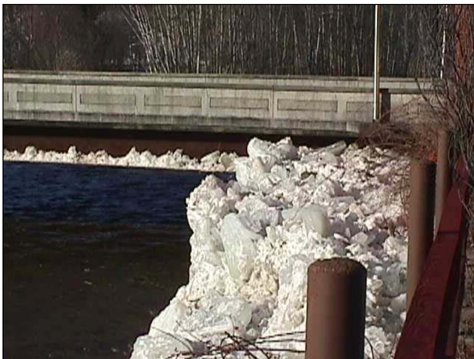
Figure 15. Upstream view of the Main Street Bridge after the ice jam of January 1999. (Photo courtesy of Greatnorthwoods.org, http://www.greatnorthwoods.org/lancaster/icejam19990124/1/ .)
