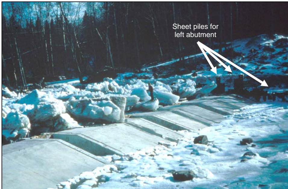
Figure 10. Ice retention upstream from the ICS during construction, winter 1980-81.
