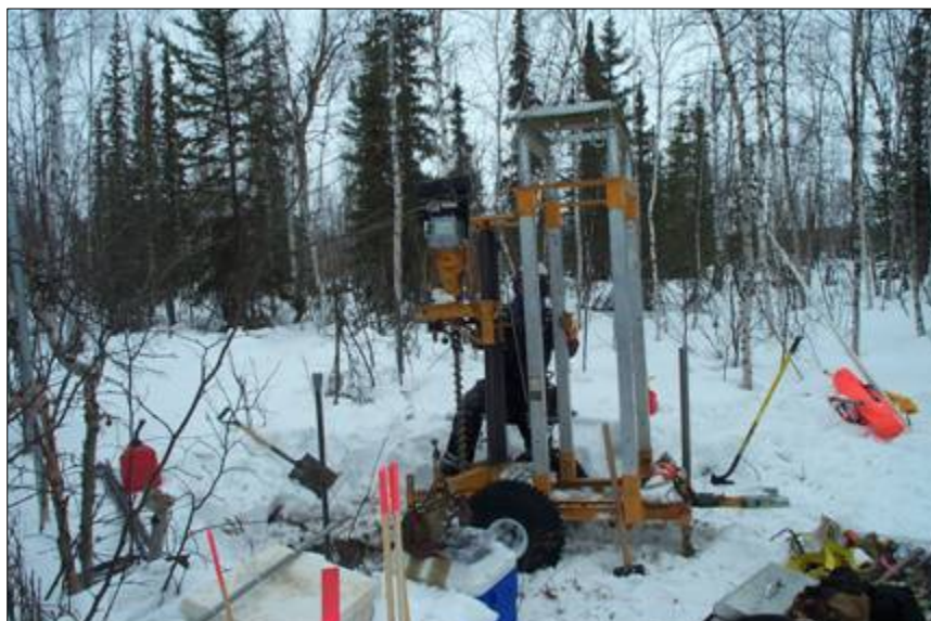
Figure 16. Drilling the well through the permafrost of Birch Island, March 2005.
