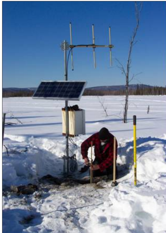
Figure 7. Installation of the new station at Murphy, March 2004.
