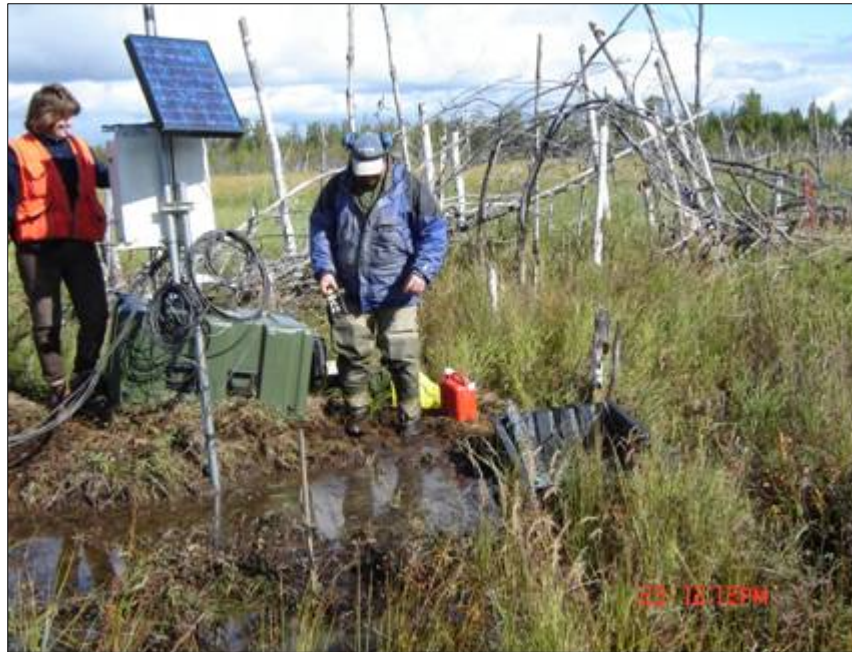
Figure 14. Upper Degraded Island station installation, August 2006.
