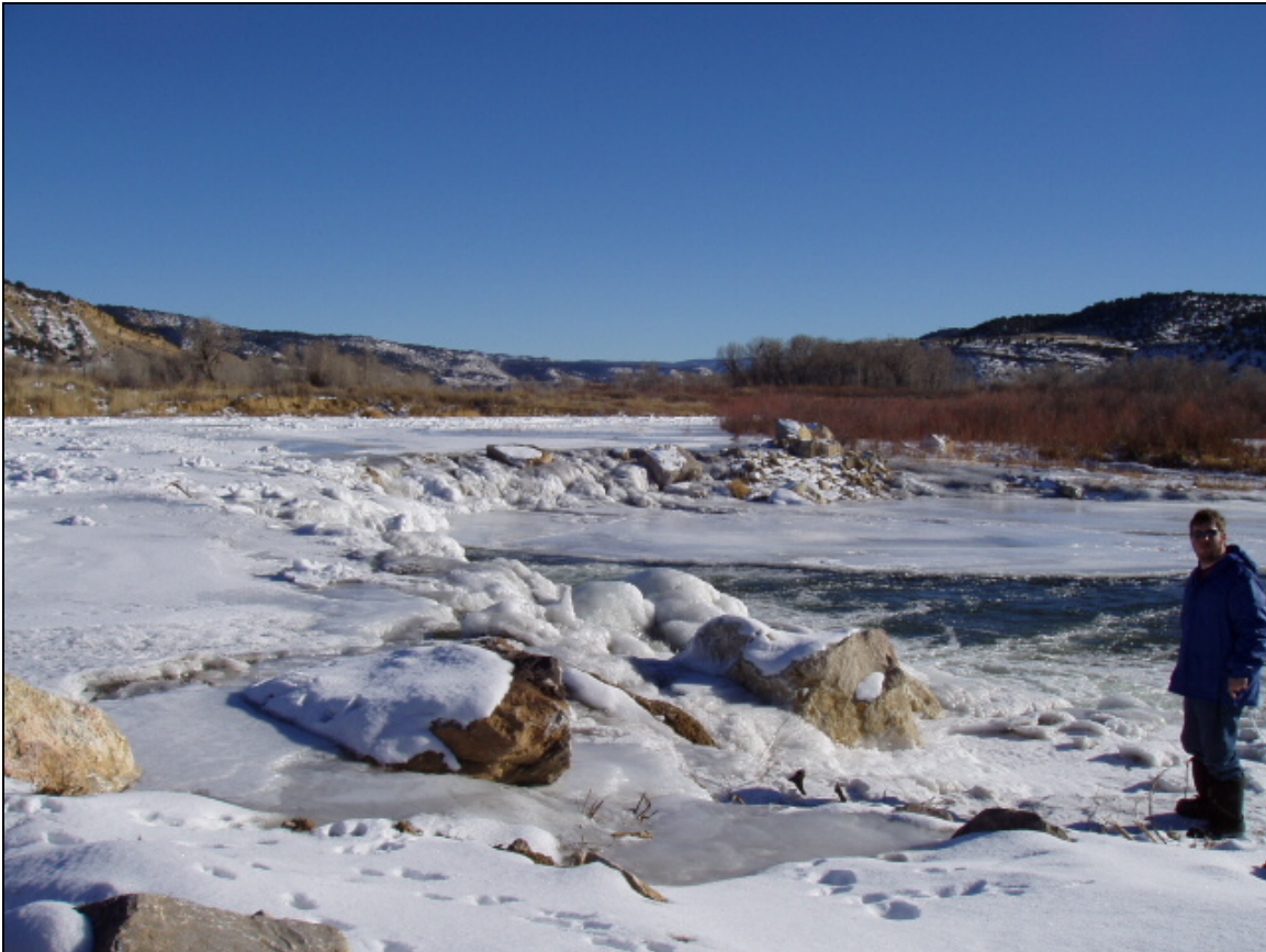
Figure 6. Freezeup ice jam at Rio Blanco diversion weir on the White River in Colorado.
