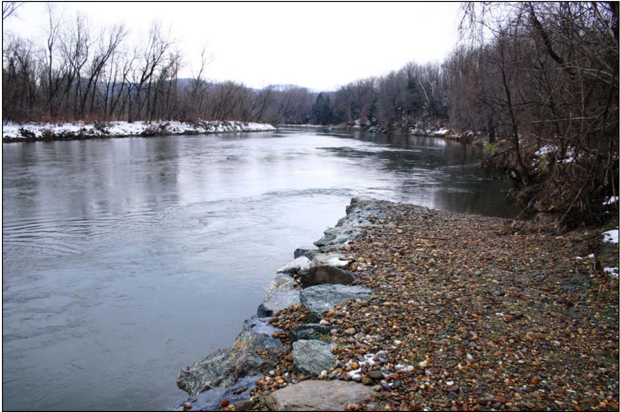
Figure 12. NRCS ice-resistant bank stabilization vane in Winooski River near Richmond, Vermont.
