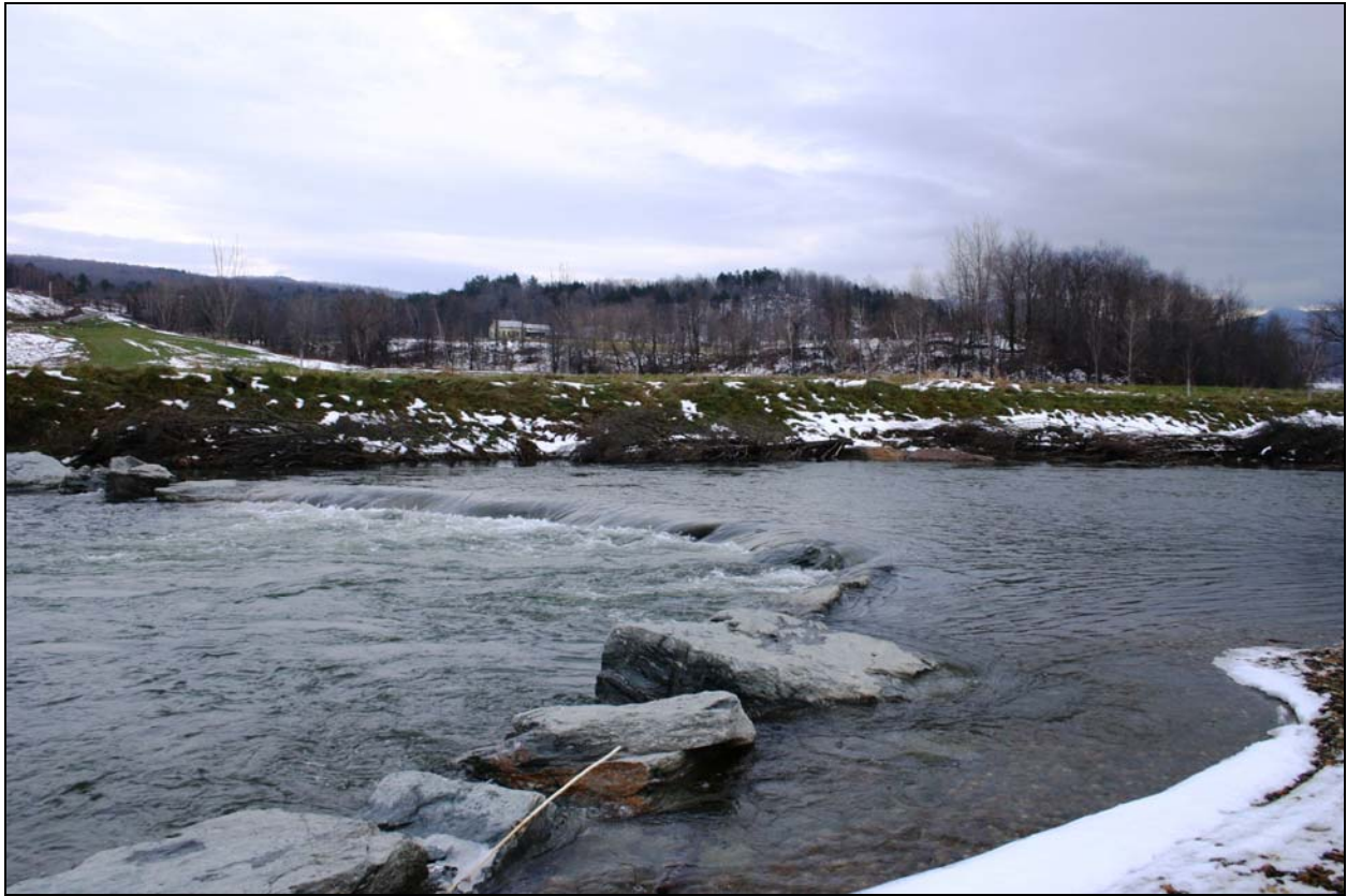
Figure 2. Rock weir on the Trout River in Vermont.
