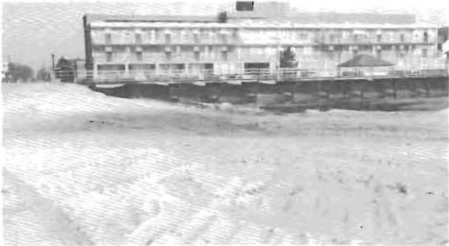
Figure 40. Borrow site under Boardwalk at Richmond Avenue on 9 March 1979. Note amount of sand removed by comparison to sand still evident behind and under Boardwalk (compare also to Fig. 39).
