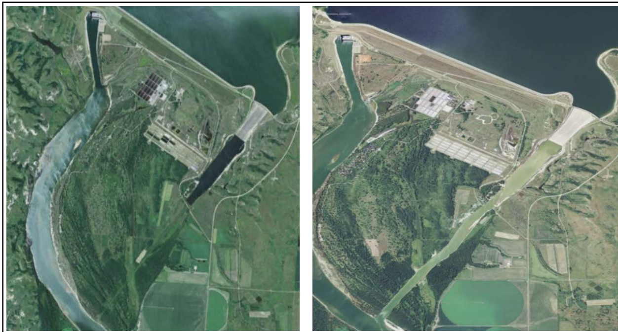
Figure 6. Garrison Dam spillway channel before (left) and after (right) the 2011 flood.
