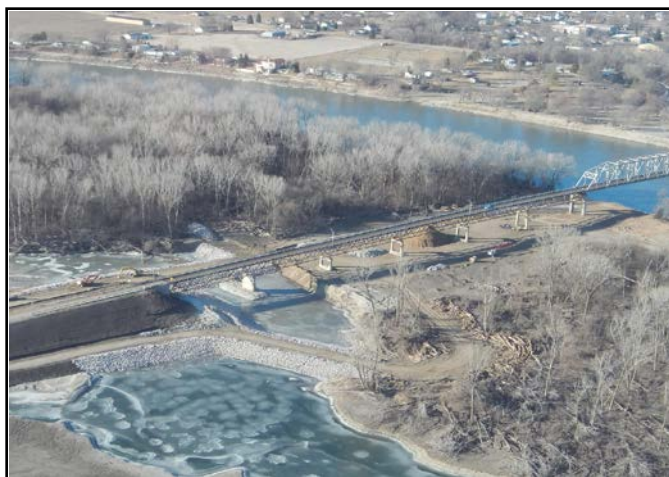
Figure 5. Bridge abutment repair at Highway 175 bridge, Decatur, NE.
