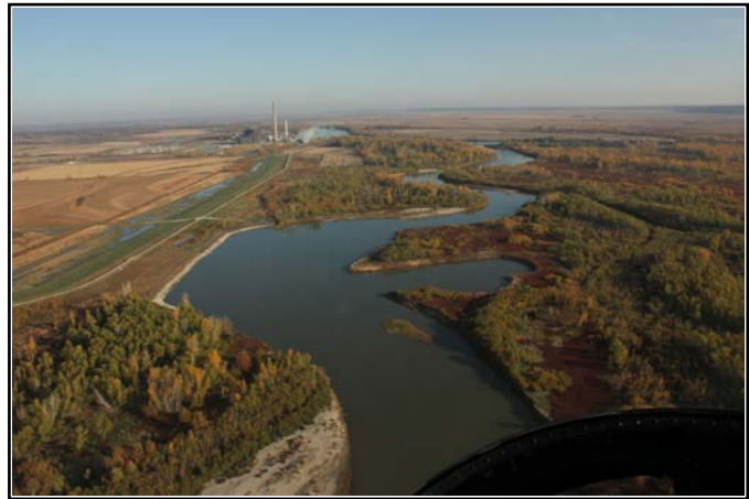
Figure 4. Repaired Upper Hamburg Bend Chute, Missouri River.
