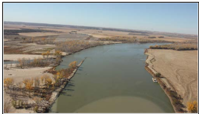
Figure 7. Lower Decatur Bend, Missouri River, revetment erosion.
