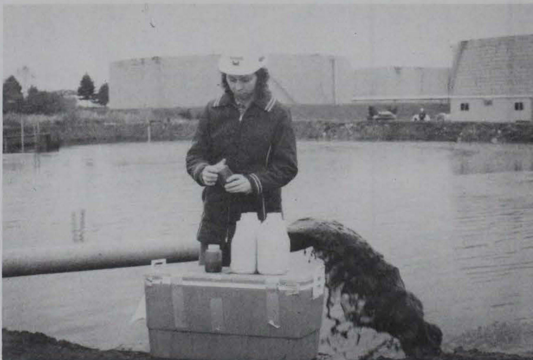
Figure 25. Influent pipe, Black Rock Harbor field evaluation
