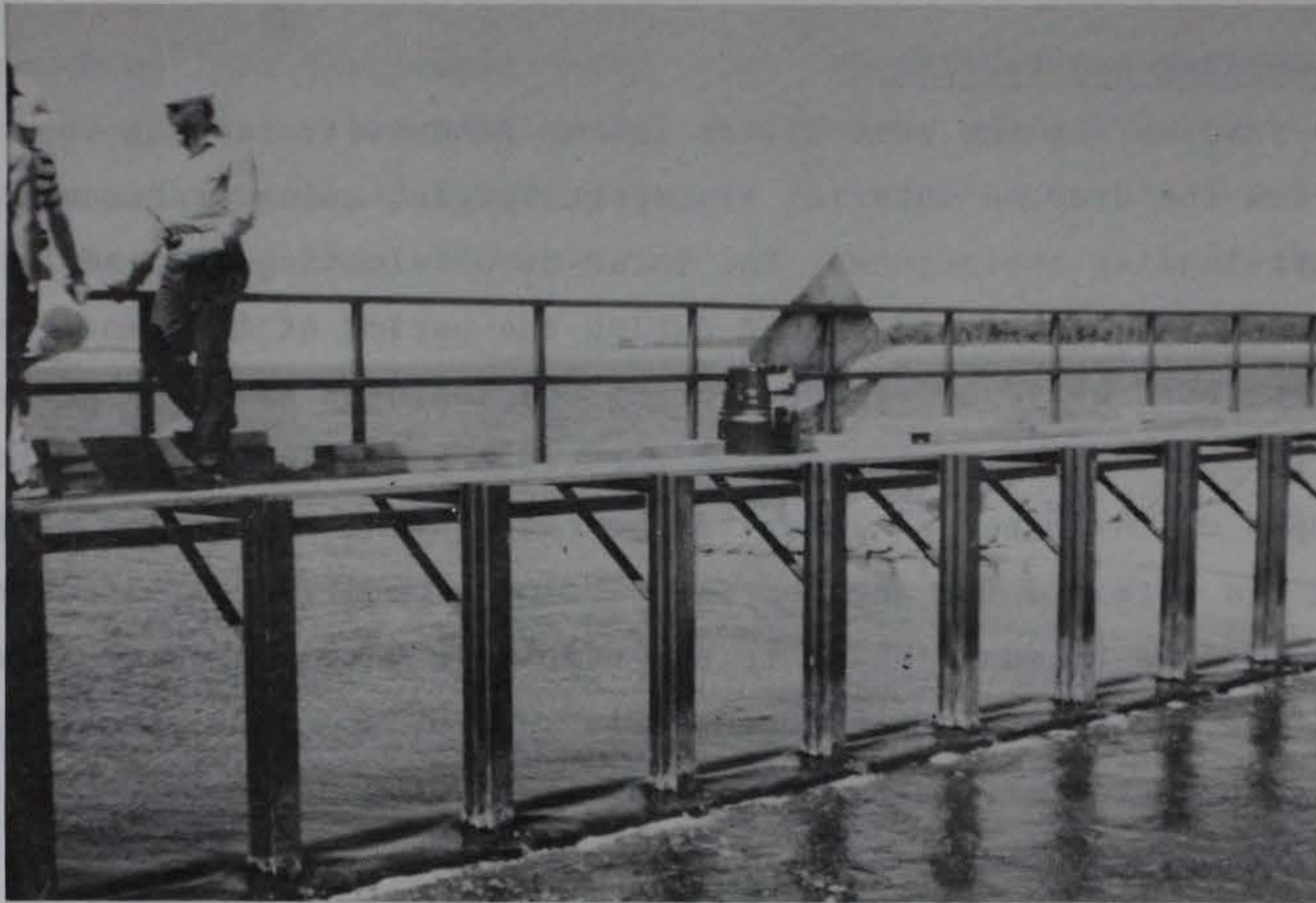
Figure 32. Fixed-elevation weir in cross dike, Hart Miller Island field evaluation
