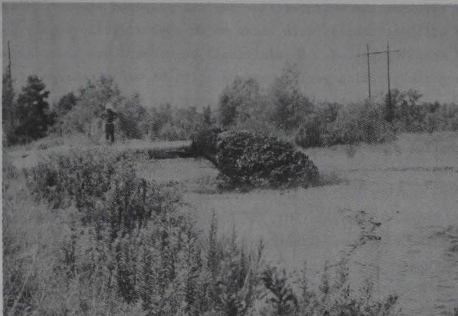
Figure 5. Influent pipe, Mobile Harbor field evaluation
