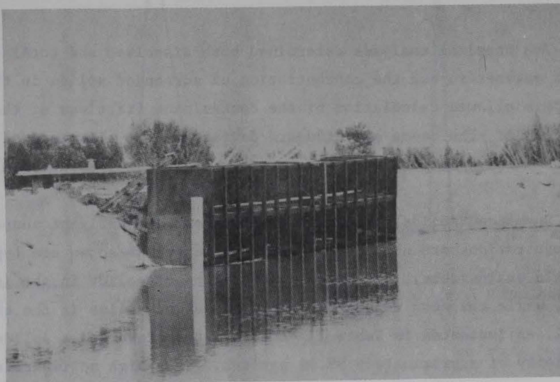
Figure 6. Box weir structure, Mobile Harbor field evaluation
