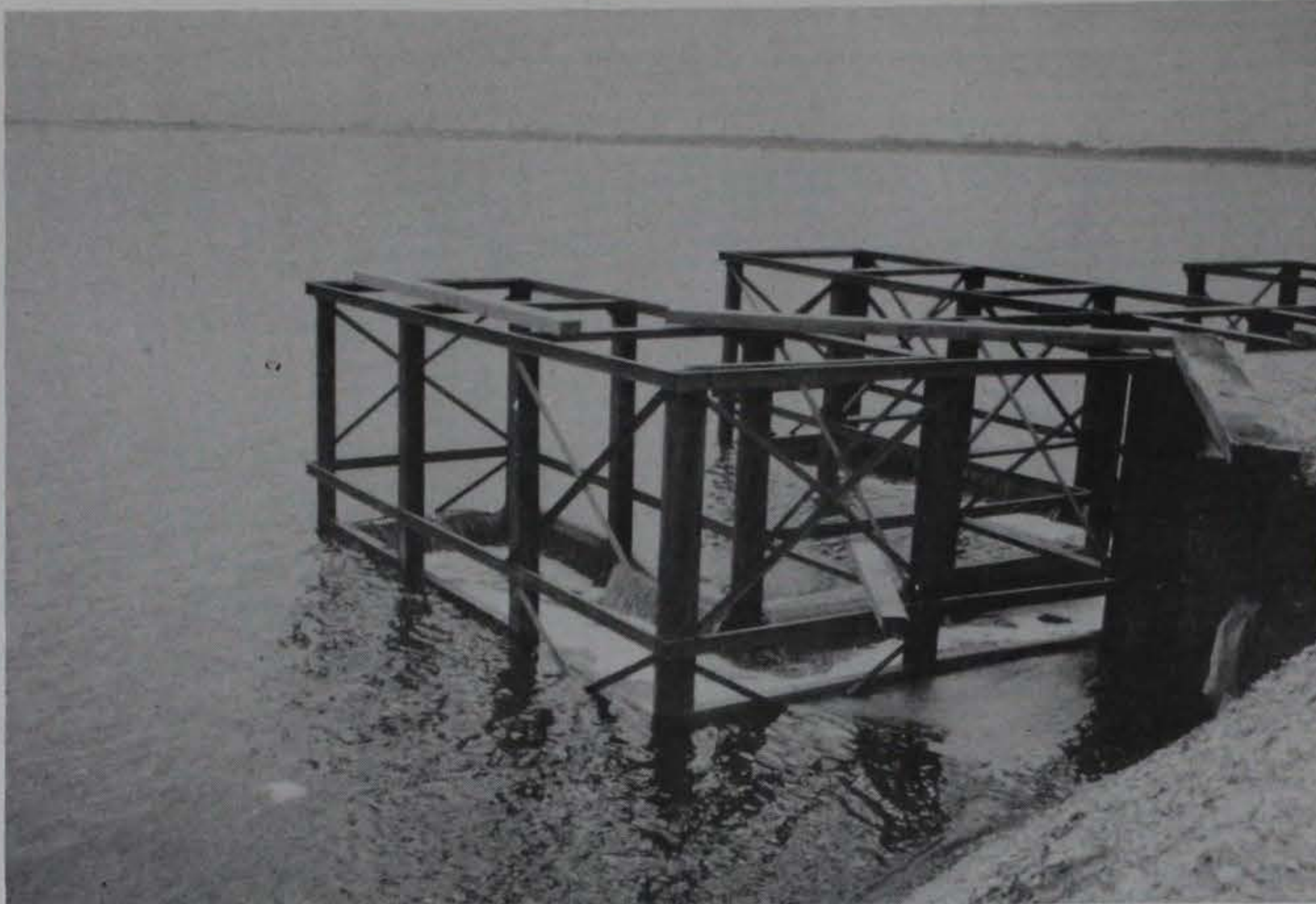
Figure 18. Polygonal weir, Norfolk Harbor field evaluation
