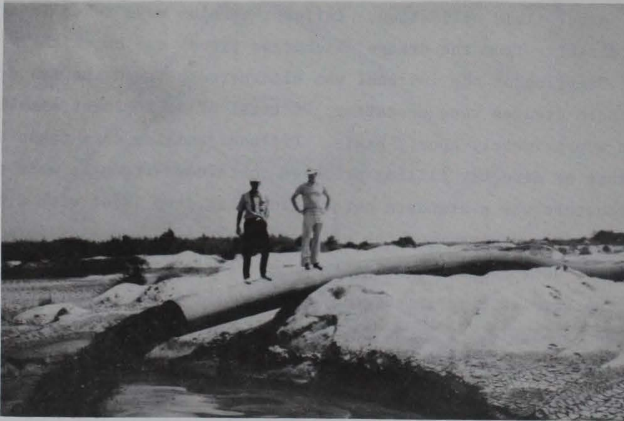
Figure 11. Dredge influent pipe, Savannah Harbor field evaluation
